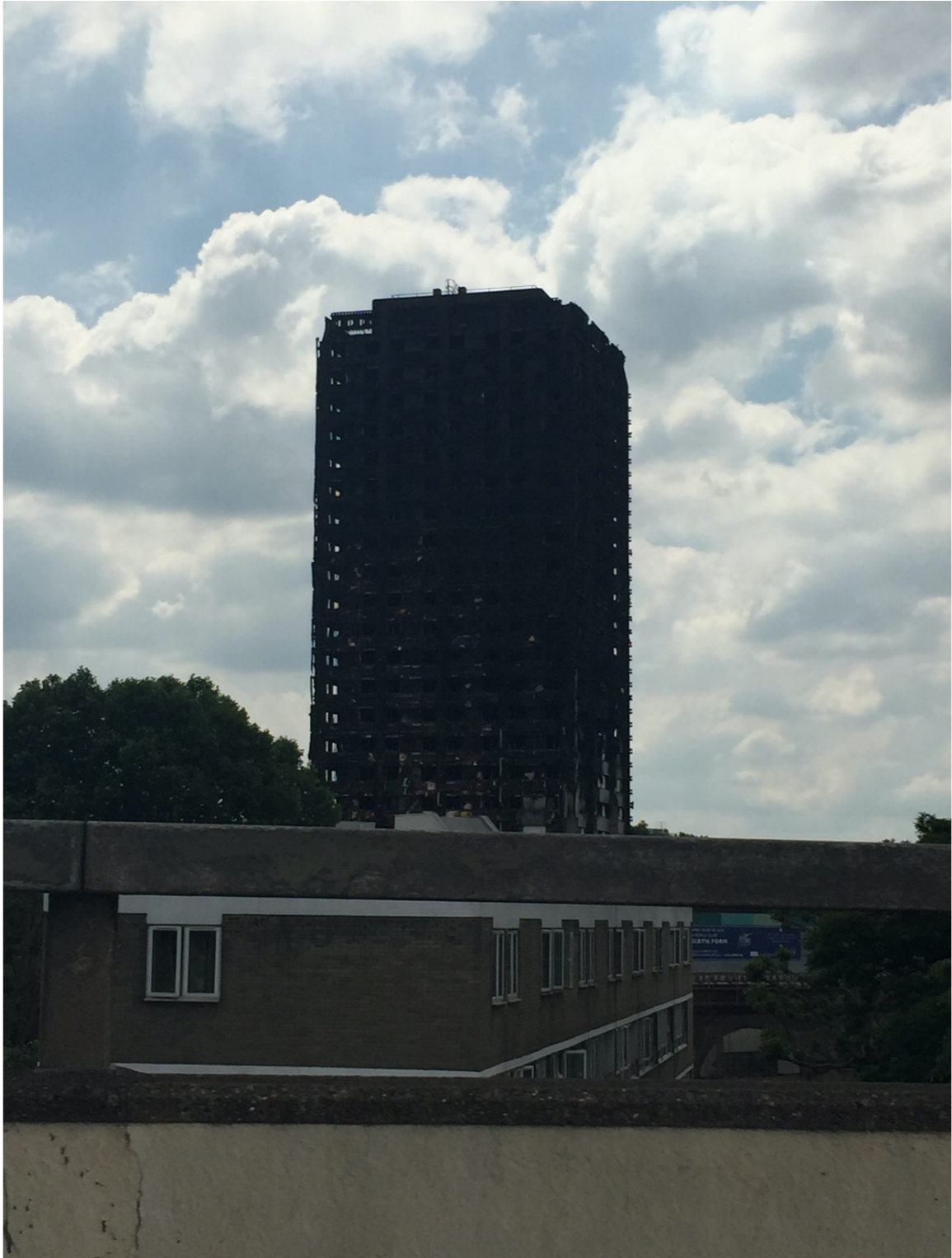
Appendix 1: Grenfell Tower, London, UK. June 18, 2017.
