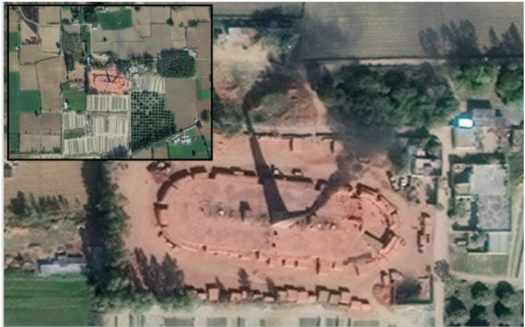
Fig. 7. An example of a Fixed Chimney Bull's Trench brick kiln @31.5385546, 75.9813821 – note the emissions from the chimney stack. From Digital Globe's WorldView-2 satellite system; pan-sharpened natural colour at 50 cm resolution; captured in November 2015. (For interpretation of the references to colour in this figure legend, the reader is referred to the web version of this article.)
