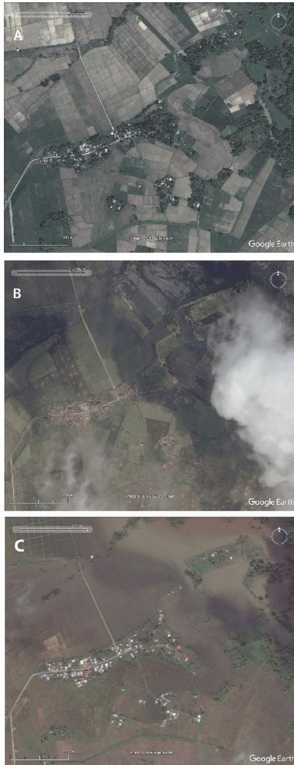
Figure 2. (A) DigitalGlobe image (23 February 2012) courtesy of Google Earth showing the community of Badiangay prior to Typhoon Haiyan. (B) CNES/Airbus image (13 November 2013) courtesy of Google Earth showing the severe wind damage to the community five days after Typhoon Haiyan passed through. (C) DigitalGlobe image (9 December 2014) courtesy of Google Earth, showing the extent of flooding around reconstructed houses following heavy rainfall associated with Typhoon Hagupit. British Geological Survey (c) UKRI 2020.
