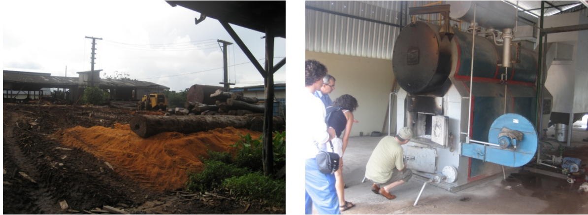
Figure 6.5: Integrated biomass utilization scheme: sawmill (left) and sawdust CHP plant (right).
