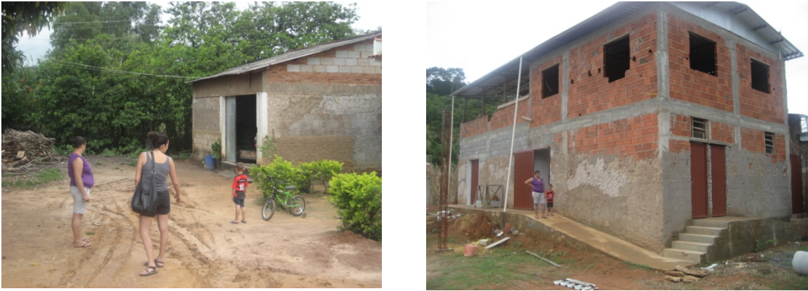
Figure 6.1: Formal sugar storage (left) and new storage and administration building (right)
