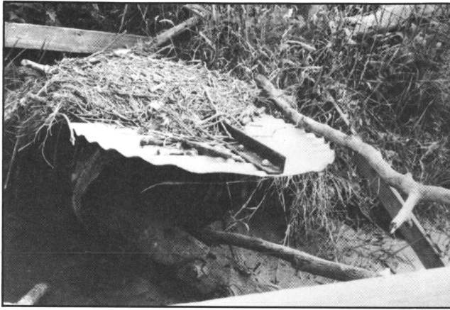
Figure 7. Remove debris from the pipe spillway inlet area.
