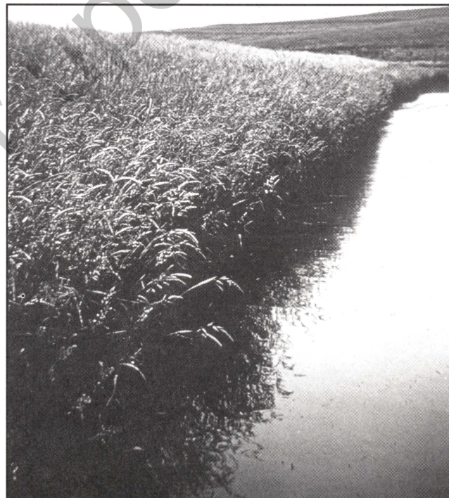
Figure 2. Fescue, reed canary or other heavy grass may be sufficient to protect the dam from wave action. To apply fertilizer annually to maintain a vigorous vegetative growth.
