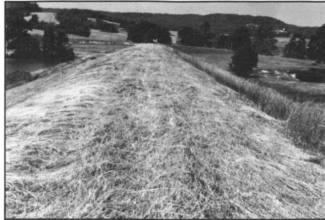
Figure 4. Keep dams mowed to help maintain an effective grass cover.
