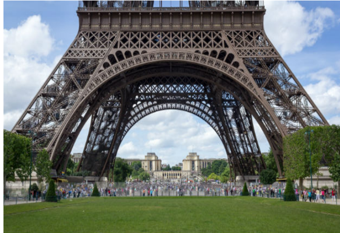
Figure 27. Detail of the Eiffel Tower showing decorative stone pedestals and decorative iron arches between the legs.
