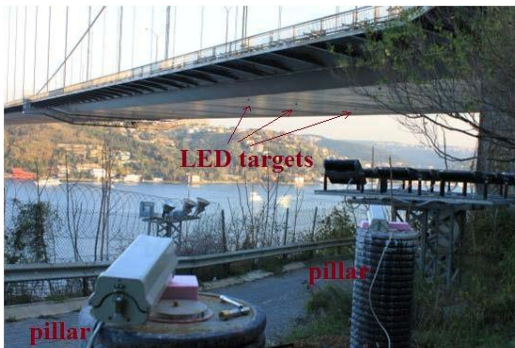
Figure 4. The two of the total four pillars
