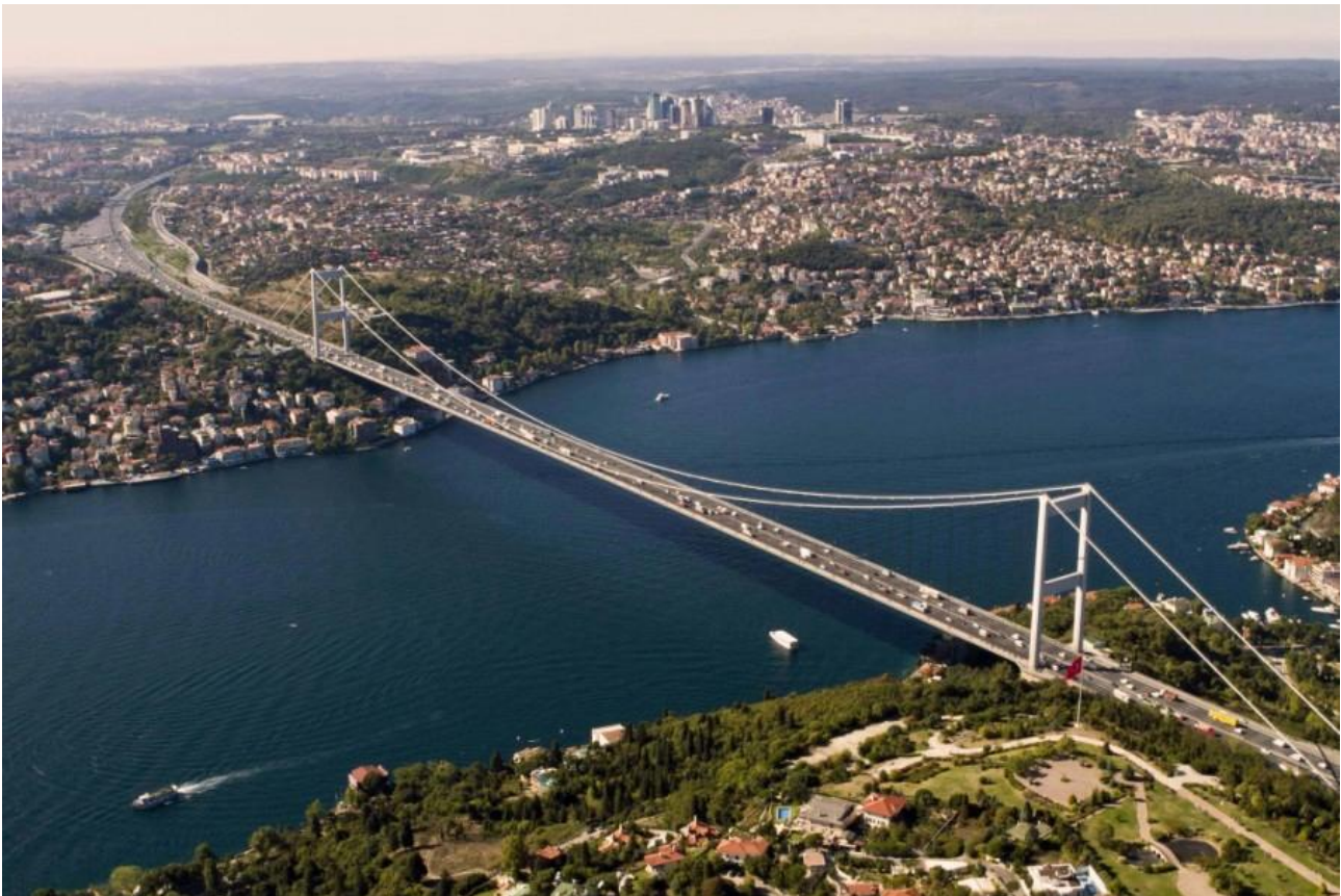
Figure 1. The second Bosphorus Bridge in Istanbul
