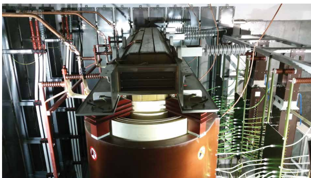
Fig. 22. Top view of a 72.5-kV, 34-MVA dry transformer located in downtown Seville. The separate on-load tap changer using vacuum switches is located on the right while the steel sheets intended to mitigate the magnetic field can be seen vertically arranged on the walls.
