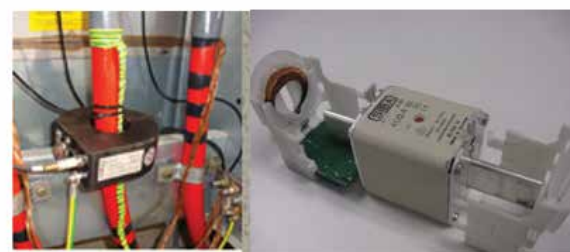
Fig. 27. Coupling system for PLC communication (left) and LV current sensor (right).
