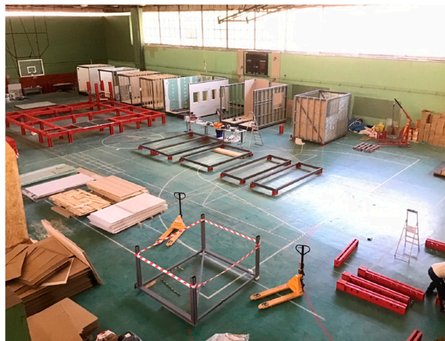
Figure 11. Aura 3.1 prototype (for SDEU19) being built in the ETSA Sports Centre and loaded onto transport. Source: SD team.
