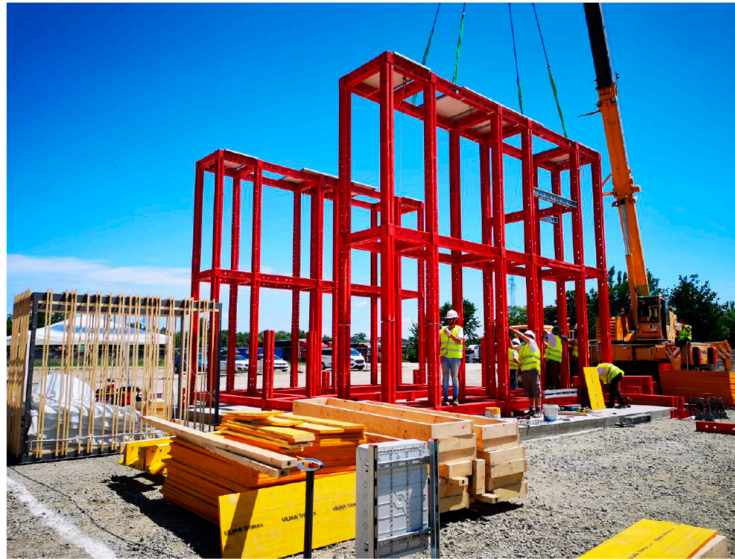
Figure 12. Assembling process of the Aura 3.1 Prototype (for the SDEU19) on the Szentendre Solar Competition site, Budapest, Hungary. Source: SD Team.
