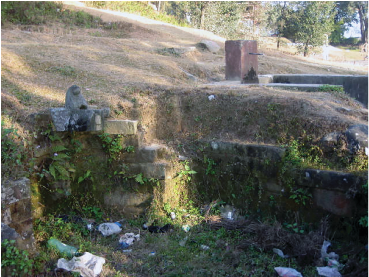
FIGURE 2. Sangdaha hiti : the traditional spout is in the left foreground; the more recent reticulated supply is in the right background.
