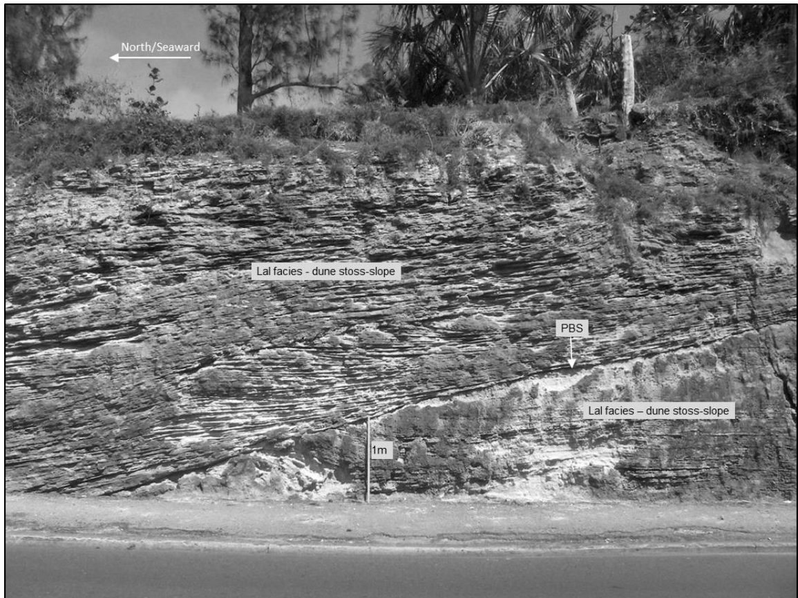
Figure 7.9. Road-cut exposure at the northern end of the Blackwatch Pass on the north shore (north and the sea are to the left). This controversial succession of Lal facies, was once believed to record the transgression of a beach onto a foredune (Bretz, 1960). Here, these deposits are interpreted as stoss-slope strata which accreted within vegetation on the windward slope of an advancing dune. The seaward-dipping prominent bounding surface (PBS) can be attributed to deflation which may have occurred during a storm. Note the projecting pinstripe laminae, above the PBS, comprising well cemented fine sand. This type of stratification which is prevalent in Bermuda's eolianites is diagnostic of inverse sorting produced by eolian climbing ripple migration. Also, compare the non-planar sub-parallel aeolian strata (Lal facies) at this locality with the planar parallel water-lain strata (Lapl facies) typical of a beach face shown in Figures 3.1.b and 7.6.
