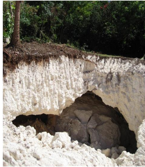
b. Cave at Lolly's Well exposed by excavation. Note interior breakdown blocks (not related to excavation) and the thin cave roof, which has progressively collapsed from below.
