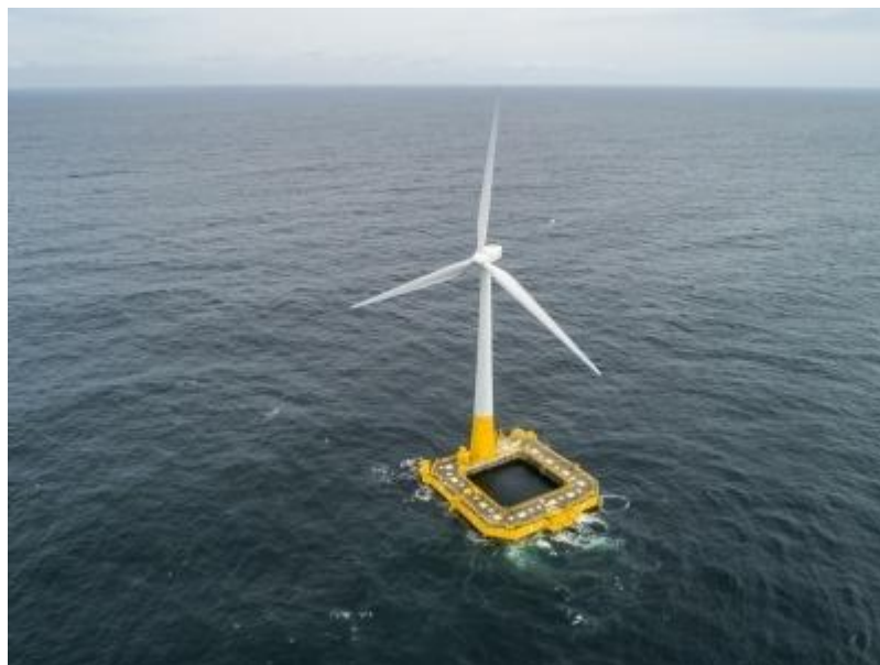
Figure 45: Ideol's damping pool structure [65]
