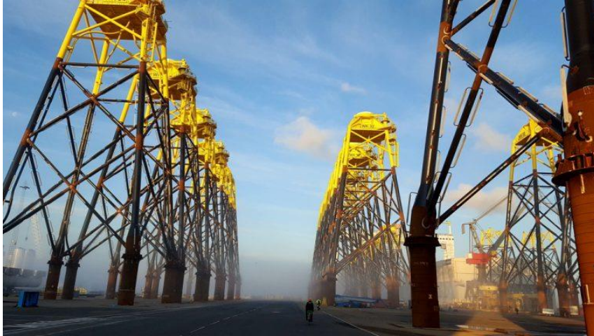
Figure 6: Jacket foundations for the Wikinger wind farm [8]
