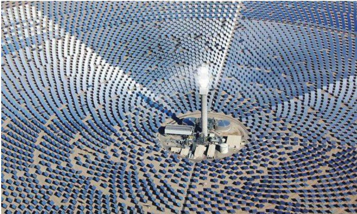
Figure 33: Concentrating solar power plant [50]
