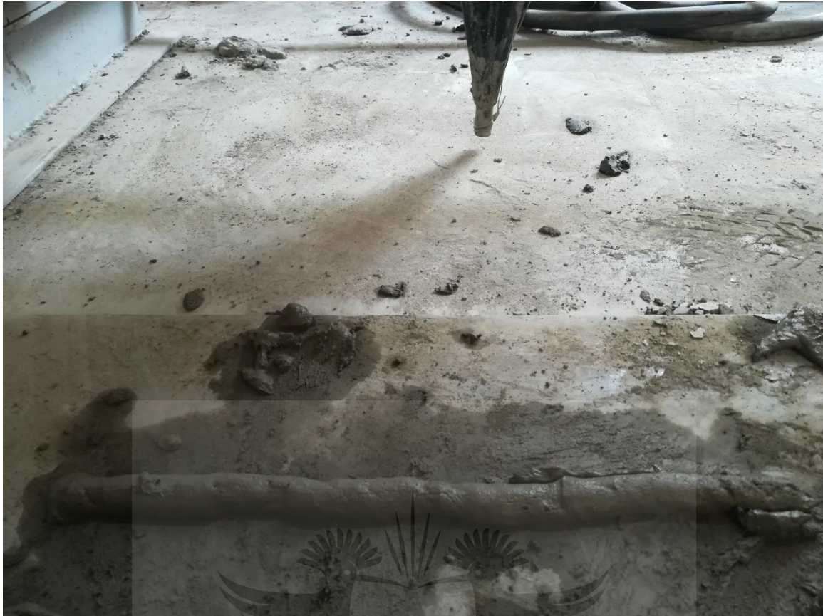
Figure 4.17: Continuous printed strip using the revised mix
