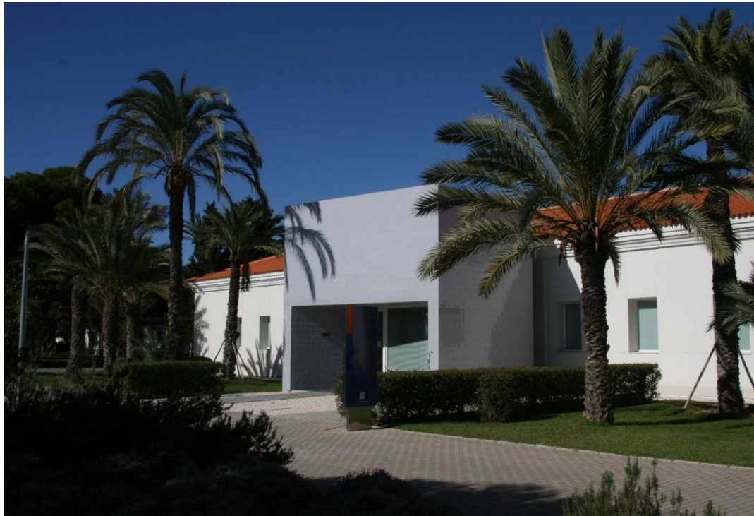
Figure 2. Faculty of Education of the University of Alicante (FEUA). Access cube covered with ceramic pieces.
