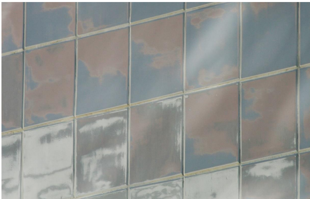
Figure 3. FEUA. Chromatic range of light reflection and iridescence in ceramic tiles.
