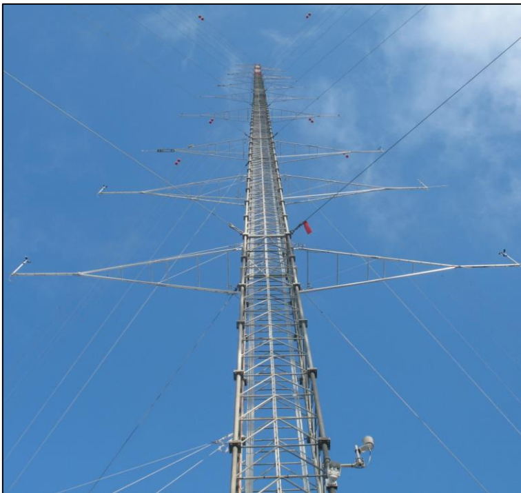
Figure 6.1: 200 m wind measurement mast at the complex terrain test site “Rödeser Berg” of Fraunhofer IEE.
