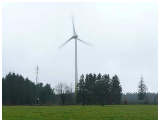
Figure 5. Enercon E33 Wind turbine
