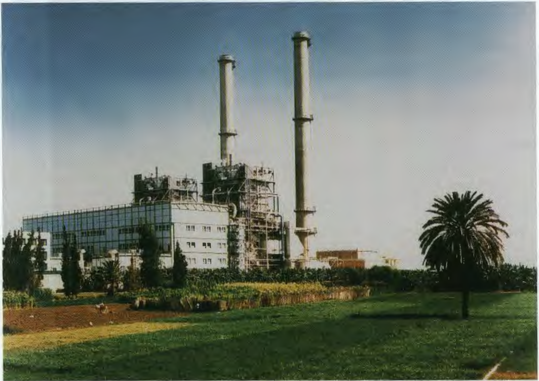
The Cairo West Power Station Extension Project, aimed at increasing electricity generation capacity, and using natural gas as a substitute for exportable oil and petroleum products.
