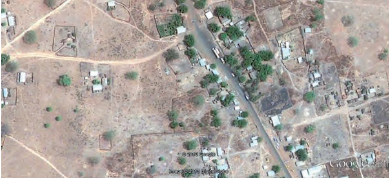
Figure 6 Google Earth image: Road surface change – tarmac to dirt – indicating boundary
