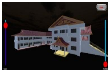
Figure 37. : Hall, Library and Laboratory Building
