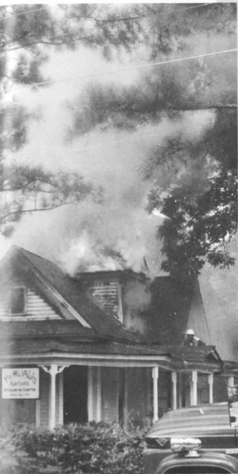
The Phi Mu Alpha house is gutted by fire.
