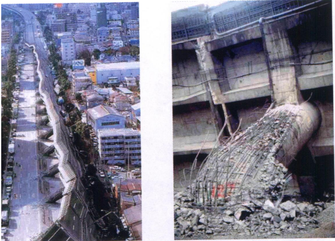
Figure 2.1 A failure in a concrete column in the 1995 Hanshin earthquake in Japan. [2]
