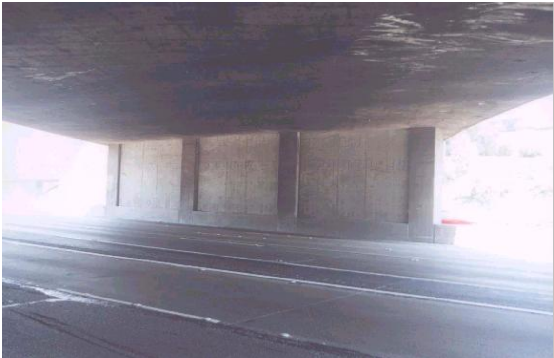
Figure 2.2 Sample bridge frames strengthened by infill walls in the Los Angeles
