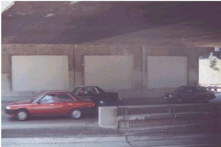
Figure 1.4 Sample bridge frames strengthened by infill walls in the Los Angeles area. [3]
