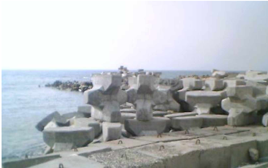
Figure 17: Breakwaters in Alexandria
