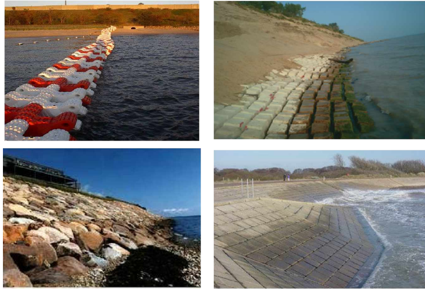
Figure 55: Floating Breakwater ( Up Left ), Beach Revetment ( Up Right ), Rock Breakwater ( Down Left ), and Concrete Canal Revetment ( Down Right )
