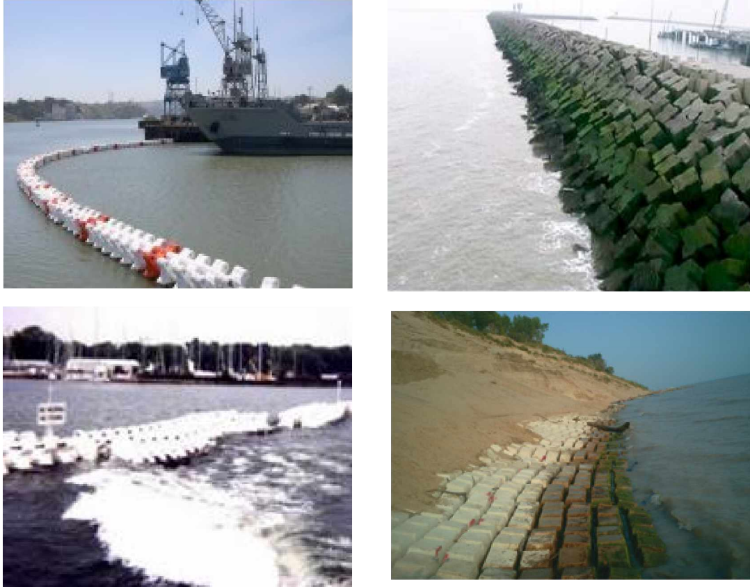
Figure 16: Photos of Floating Breakwater ( Left ) and Revetment ( Right )
