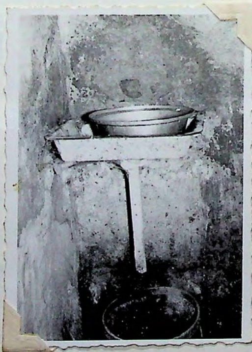
"... it has running water, but without drainage...."
