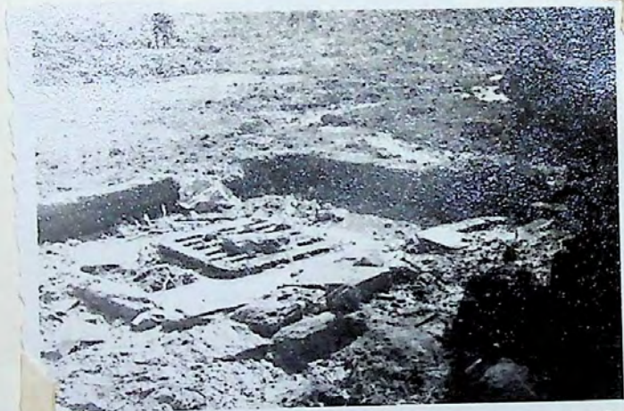
One of the inspection chambers in the Ezab, into which the drainage car empties its content after being filled.
