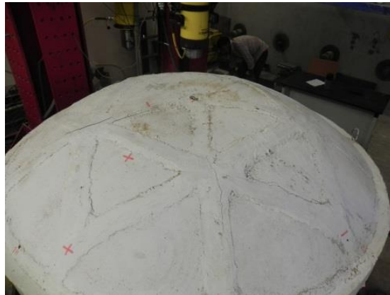
Fig. 181: Cracking pattern of the experimental model
