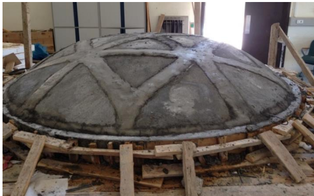
Fig. 99: Grouting of inter-panel joints
