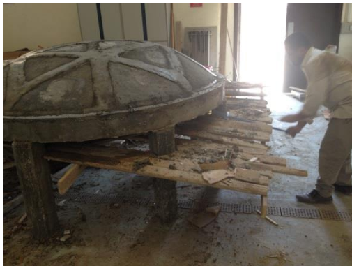
Fig. 100: Demounting of all formwork and scaffolding
