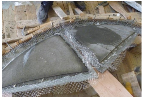
Fig. 94: Plywood sheet placed in between panels to overcome dimension discrepancies
