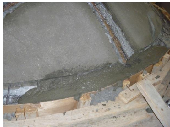
Fig. 98: Casting of top 2 cm of the ring beam (Part B)
