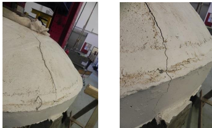
Fig. 185: Transverse crack in the ring beam
