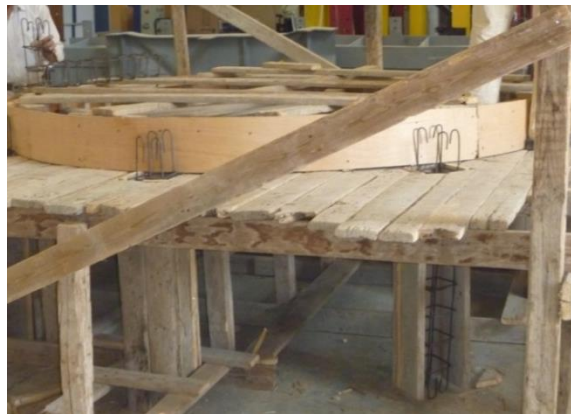
Fig. 77: Placement of column reinforcement cages
