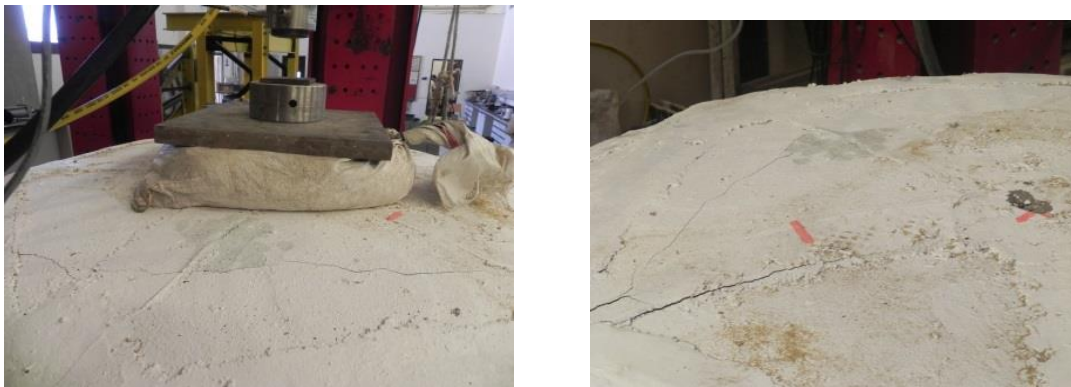
Fig. 184: Cracks in the imperfect panel
