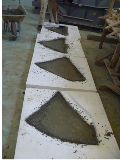
Fig. 85: Panels cast without reinforcement insulation
