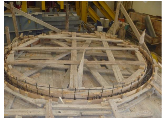
Fig. 79: Ring beam dowels
