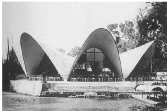
Fig. 2: Los Manantiales restaurant by Felix Candela ( www.structurae.co.uk )
