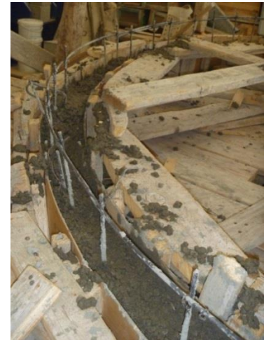
Fig. 81: Casting of part A of the ring beam
