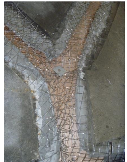
Fig. 96: Straightening of wire mesh reinforcement
