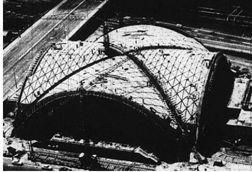
Fig. 5: 1977 barrel vaulted roof of concrete triangular panels [1]
