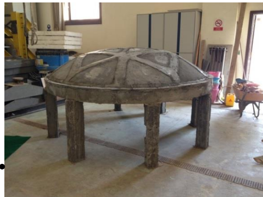
Fig. 100: Demounting of all formwork and scaffolding
