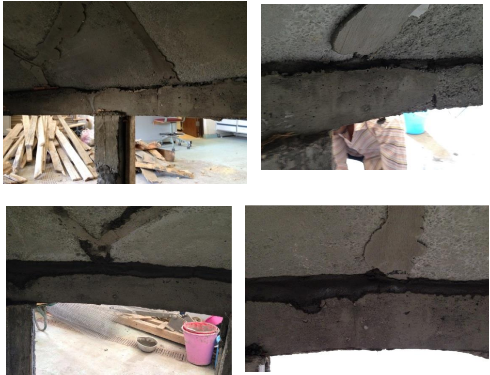
Fig. 101: Grouting of the final part of the ring beam (Part C)
