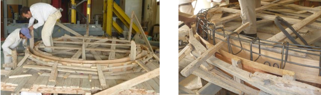
Fig. 78: Placement of ring beam reinforcement
