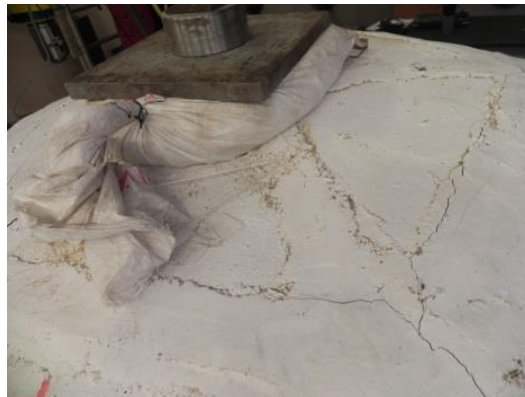
Fig. 182: Central crack of the experimental model
