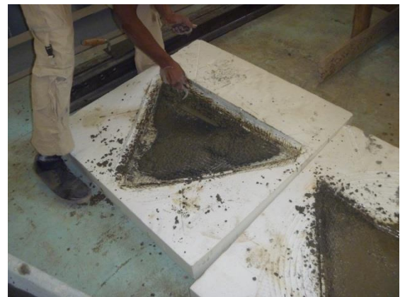
Fig. 88: Surface finishing of shell panels
