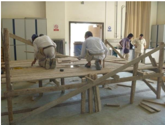
Fig. 75: Supporting frame for casting of the columns and ring beam
