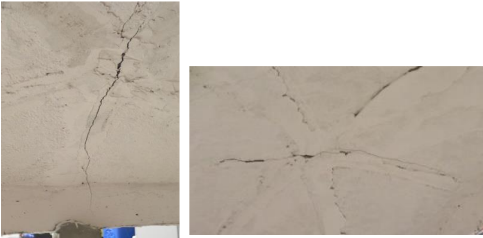
Fig. 186: Structural cracks on the lower surface of the cap
