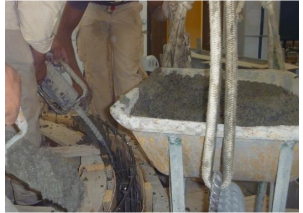
Fig. 80: Casting of columns
