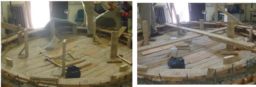
Fig. 92: Construction of scaffolding props
