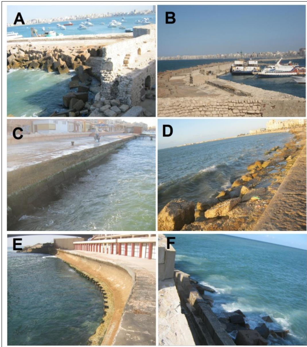
Figure 4-13: Structural inspection of non-rubble and composite structures in year 2013.
