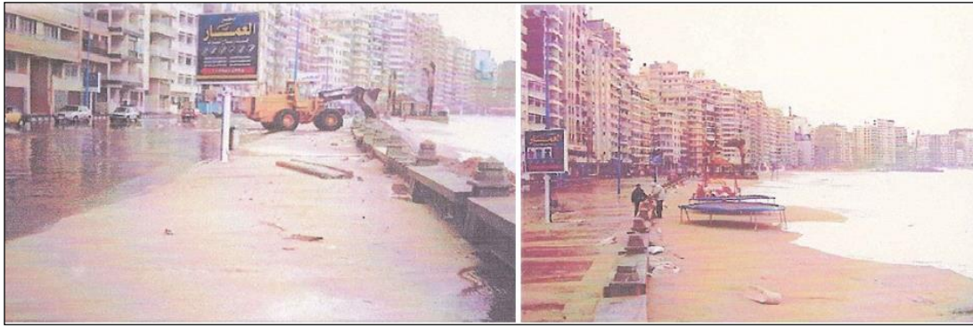
Figure 1-3: Storm surge in Al-Mandara area in 2003 (Courtesy of Arab Contractors).
