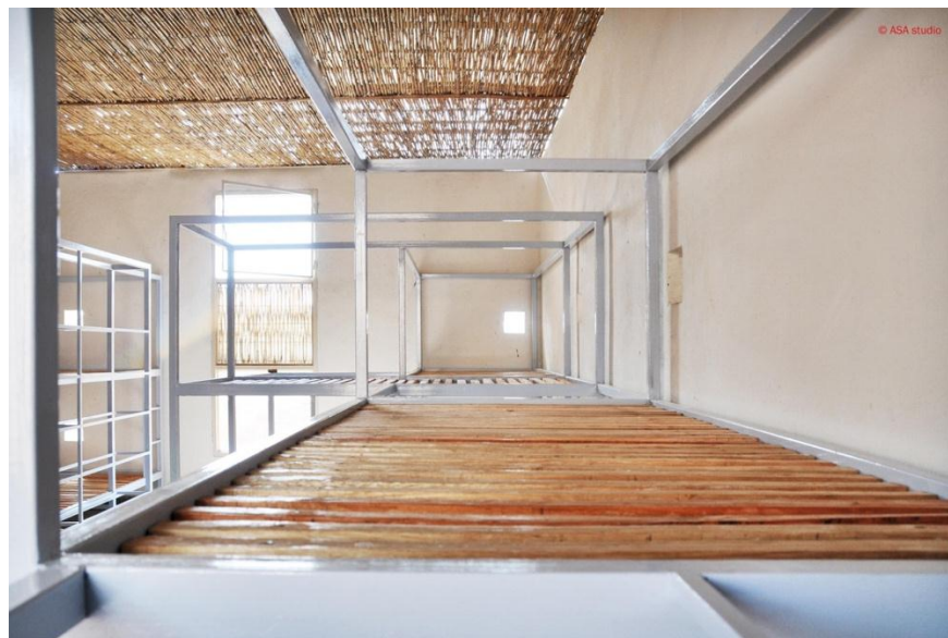
Figure 12: School Dorms Under Construction
