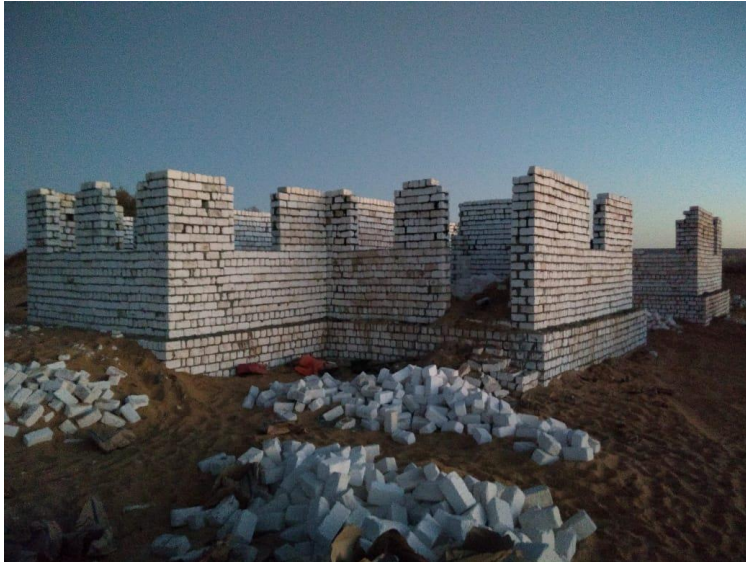
Figure 29: Dates Pack-house Under Construction in December 2018
