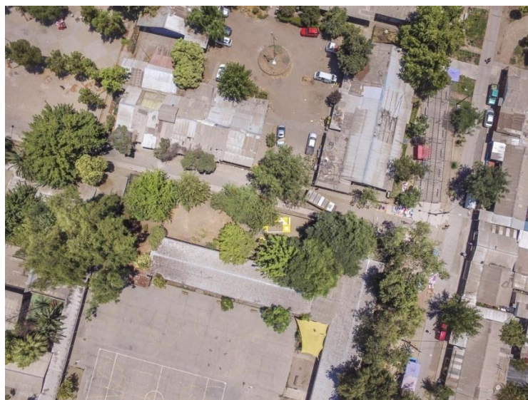
Figure 9: Playground's Site Location
