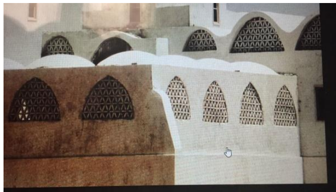
Figure 27: New Baris Market Close-up
