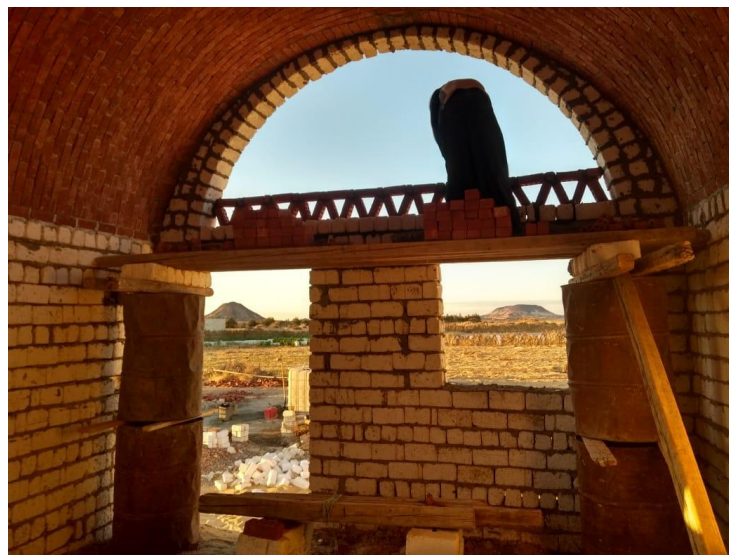
Figure 31: Interior Photo During Construction
