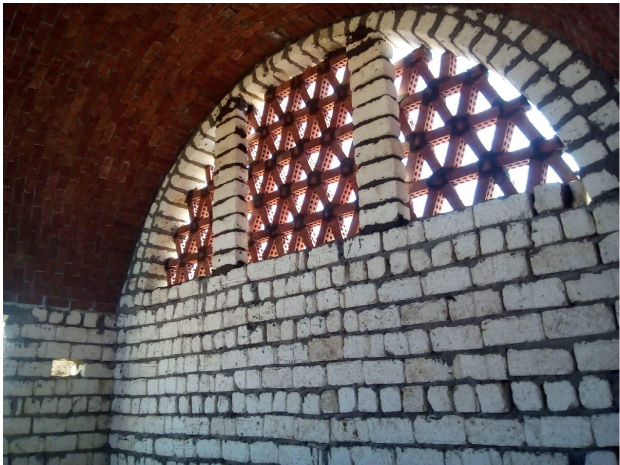
Figure 34: Vault Built with the Supports
