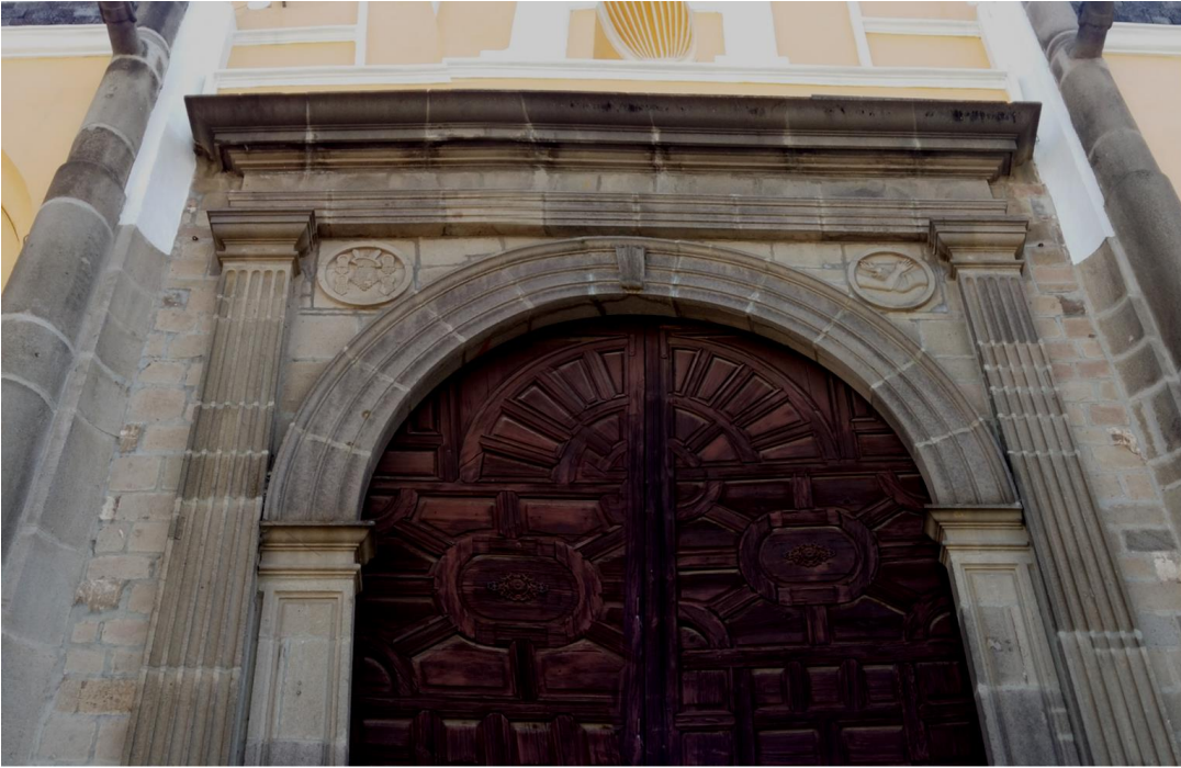
Fig. 3.28. Main gate of the Chapel with Franciscan medallions on the spandrels. Notice the different kind of masonry on the dividing columns with the gutters, and the gate.
