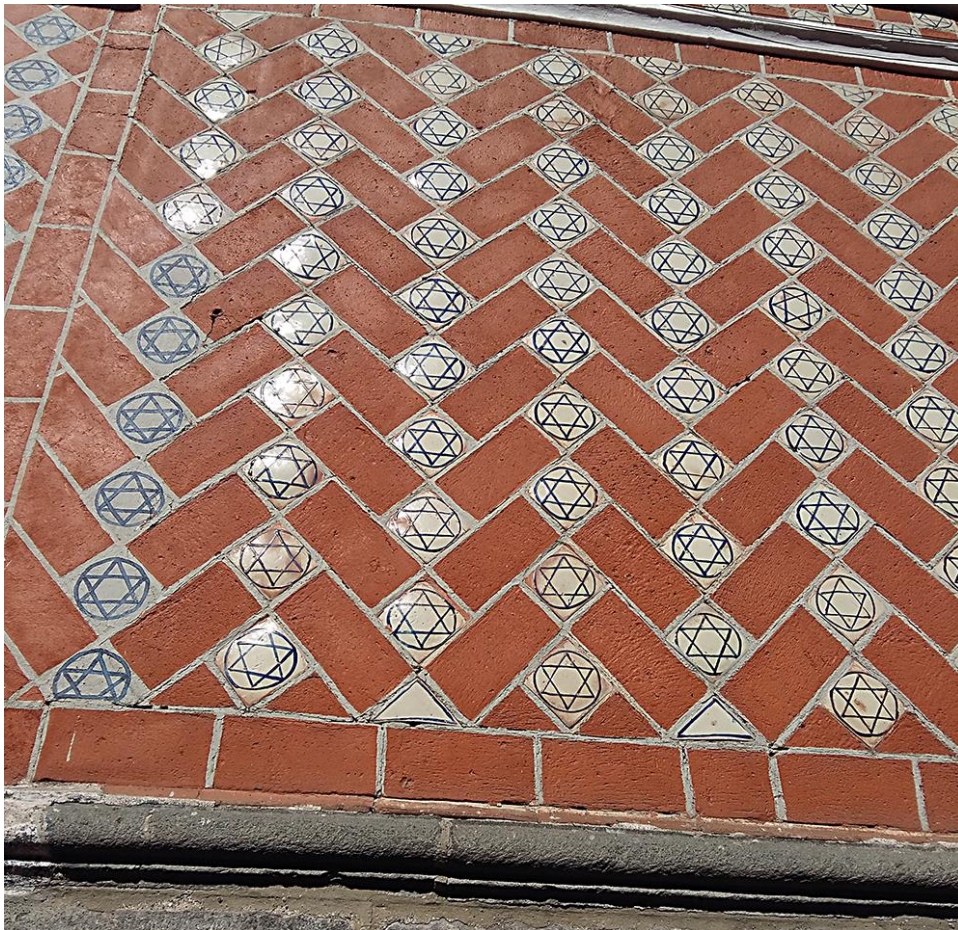
Fig. 3.34. Brick and tilework decoration on the wall of a house in Puebla. This one looks fairly new, but according to Toussaint, this is an old tradition in this city.
