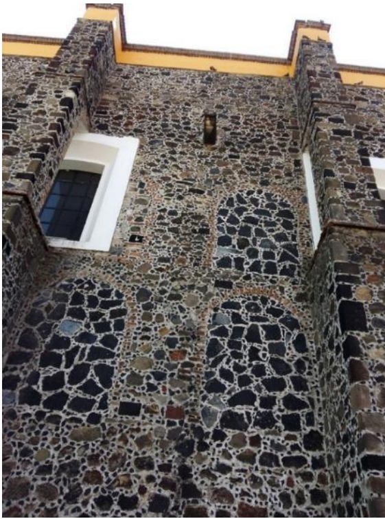
Fig. 3.30 Rear wall of the Chapel, showing sealed windows, buttresses and masonry. Source: L. Barragán
