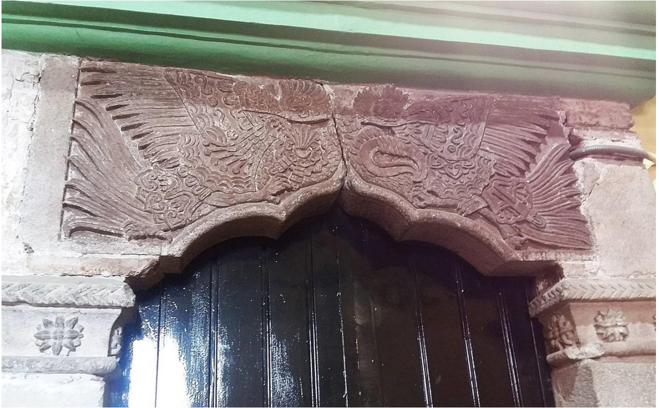
Fig. 1.36. Arcuated stone lintel in the lateral chapel in the Church of San José, Tlaxcala.
