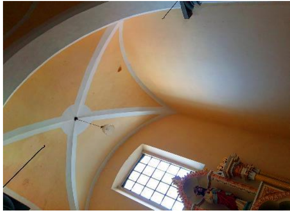
Fig. 3.23. Cross vault on side nave. Source: L. Barragán.
