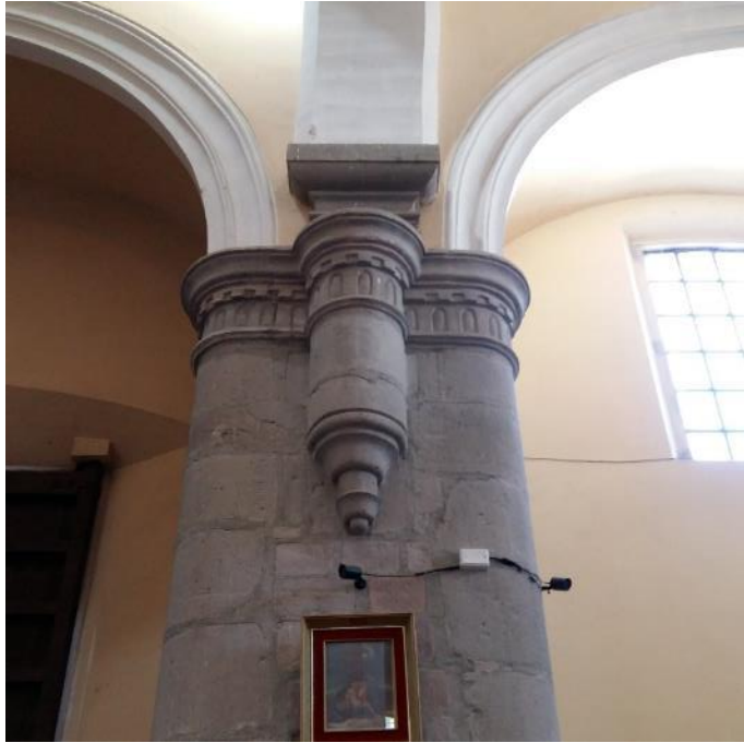
Fig. 3.17. Back of the stone pier dividing each gate.
