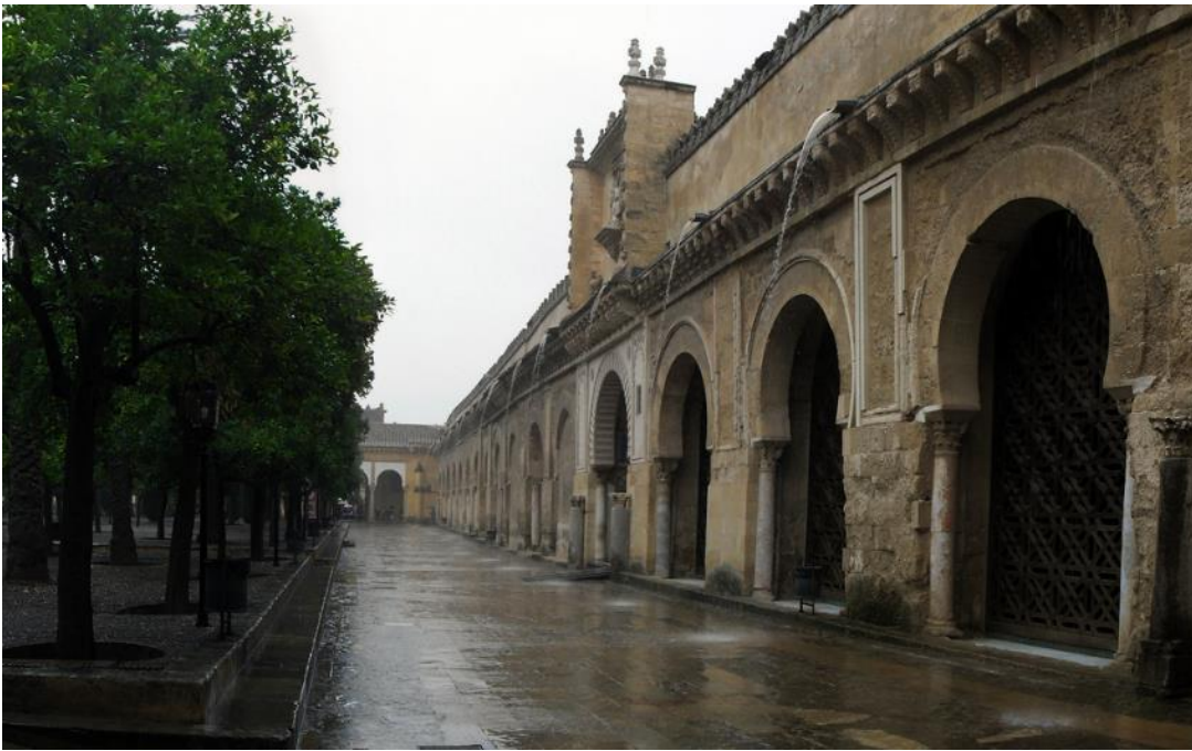
Fig. 3.29. Arcaded entrance to the Mosque of Cordoba showing frontal gutters in action.
