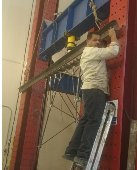
Figure 42: Installation of the Steel Beam
