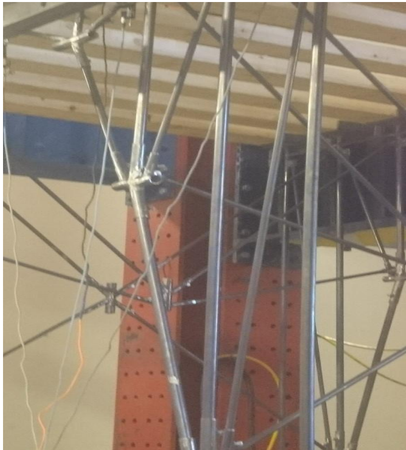
Figure 47: the Deflection at specimen #1
