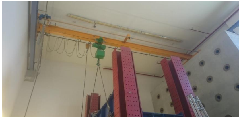
Figure 31 : the Crane used in the moving of the Beam
