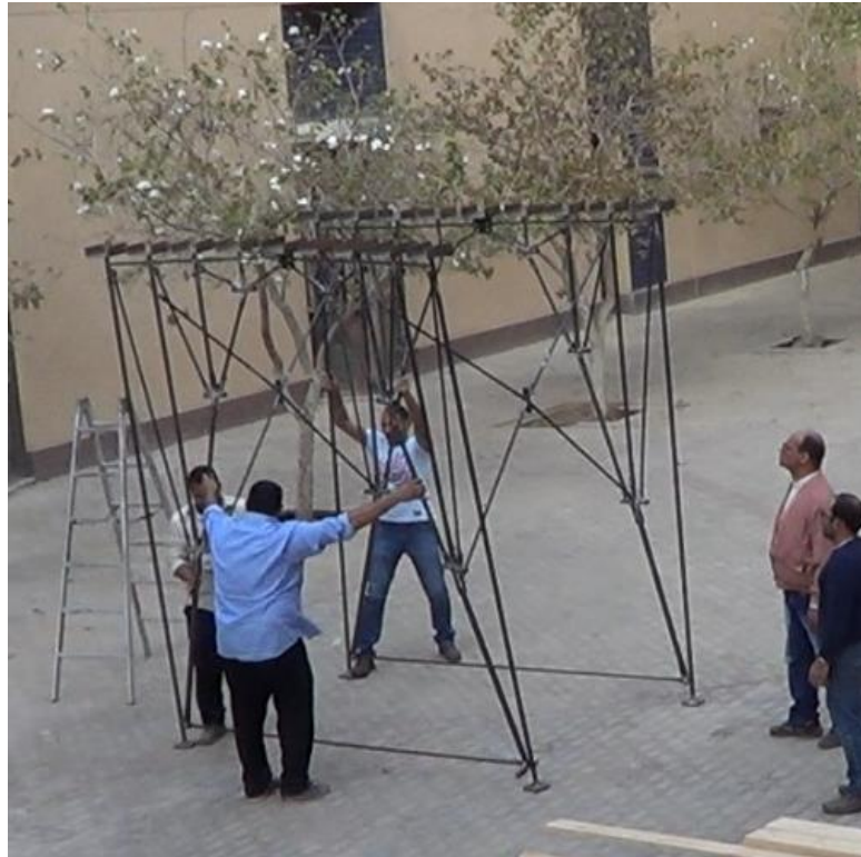
Figure 22: Erecting the Trusses
