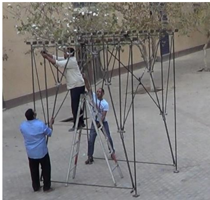
Figure 23: Connecting the bracing system to the truss using a ladder
