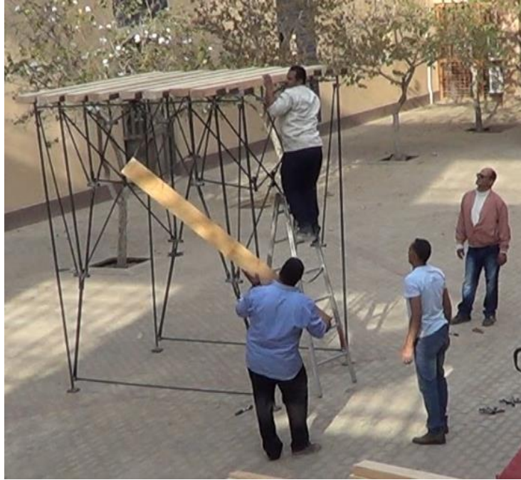
Figure 24 : The joists are put on top of the U heads
