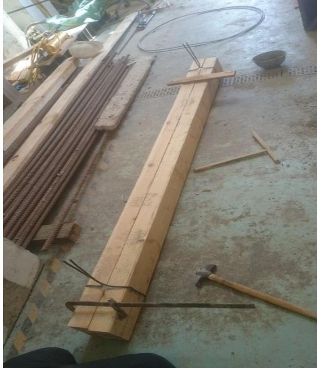
Figure 44: Connecting the two Wooden Beams
