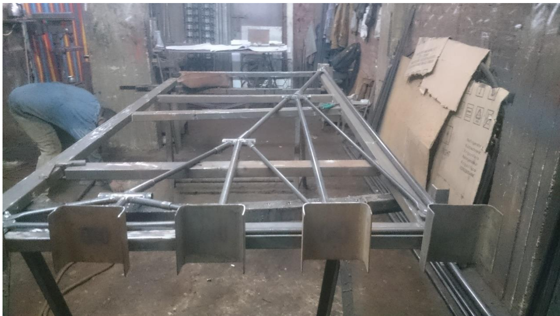
Figure 16 : Fixing the members to the Square Frame
