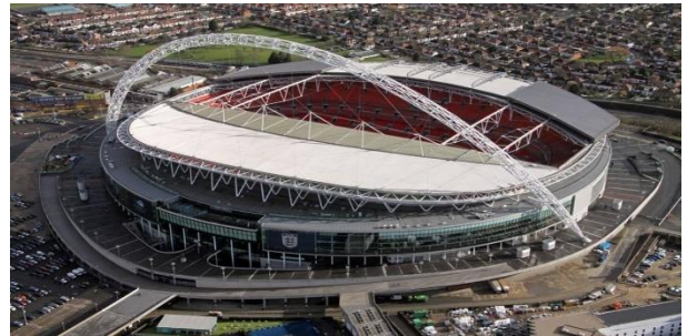
Figure (20) represents Wembley Stadium (Wembleystadium, 2017)
