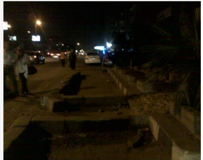
Photo (5) Encroachments by a gov. entity; No lights
