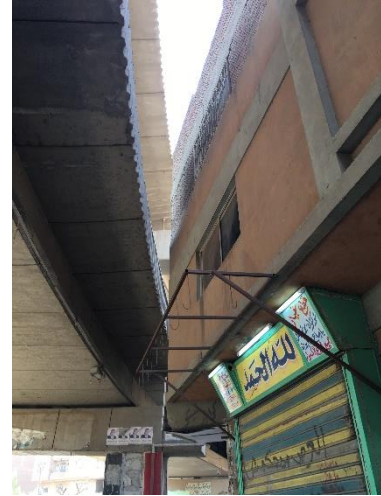
Figure 38 steel bars installed on the windows of the second floor (personal photograph by author. 24.
