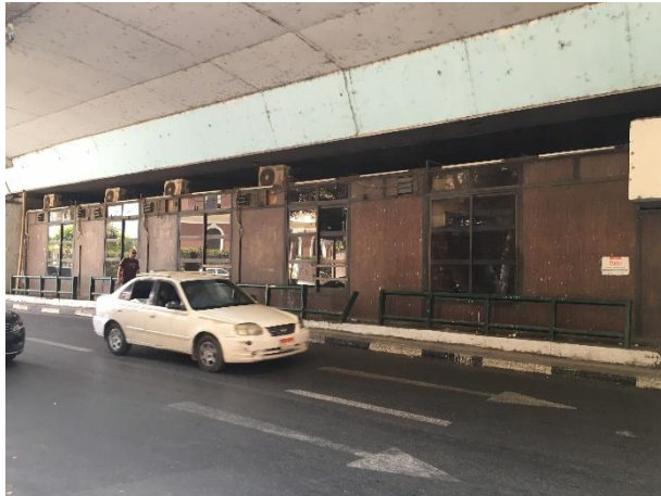
Figure 26 A mosque established under the bridge with AC units installed (Personal photograph by author. 3. Sep.2016)
