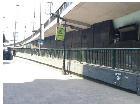
Figure 29 light structure used to close the space under the elevated road (Personal photograph by author. 3. Sep.2016)
