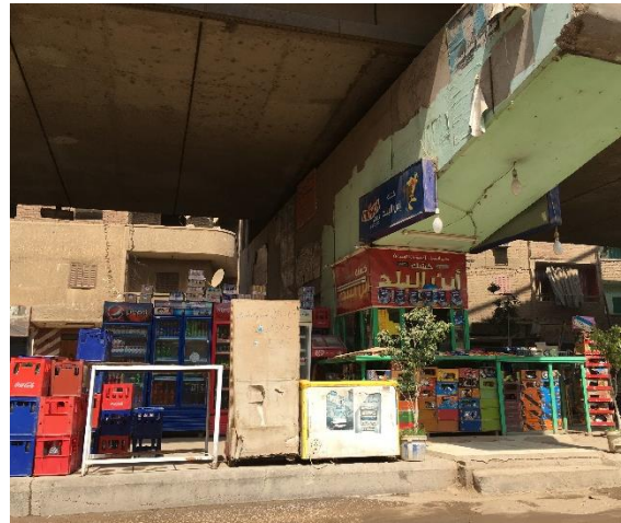
Figure 42 Kiosk in Saft El Laban integrating the corridor structure within its own structure. (Personal photograph by author. 24. Sep.2016)
