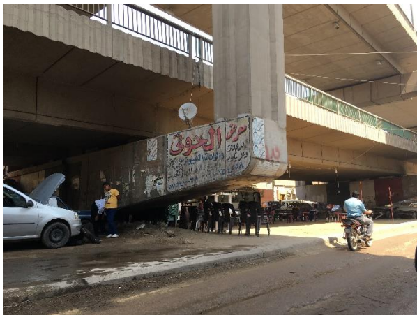
Figure 39 Car Maintenance workshop at the begging of Saft El Laban Corridor (personal photograph by author. 24. Sep.2016)
