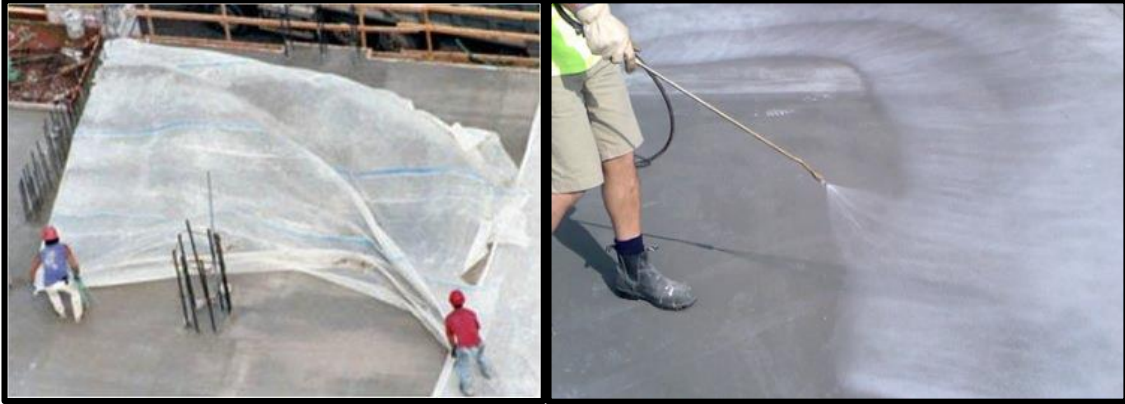
Figure 1-3: Sealed curing plastic sheeting (left) - curing compound (right) (Suryakanta, 2014)
