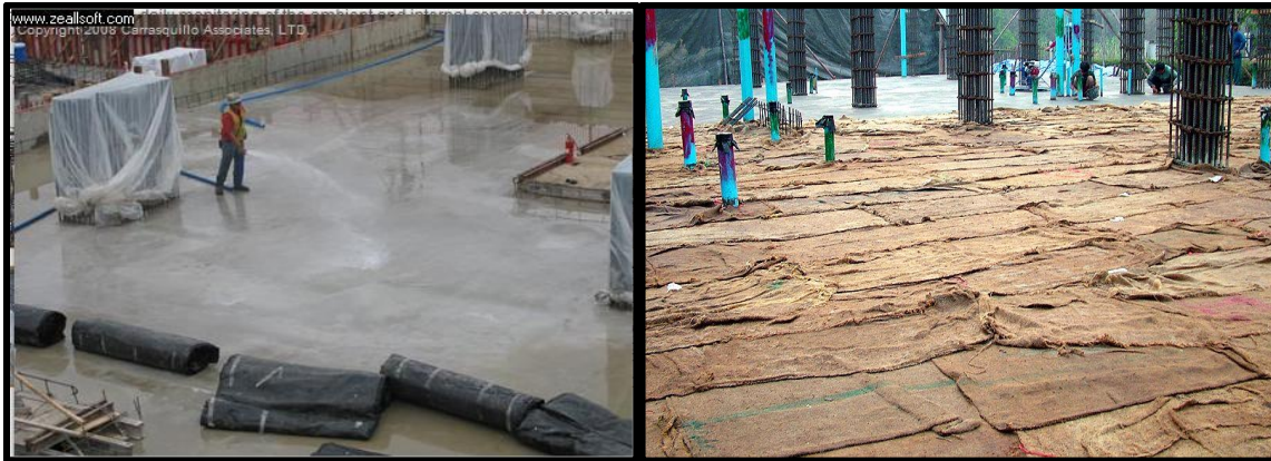
Figure 1-2: Water adding curing methods: water spraying (left) - wet burlap (right) (Foster Supply, 2012)
