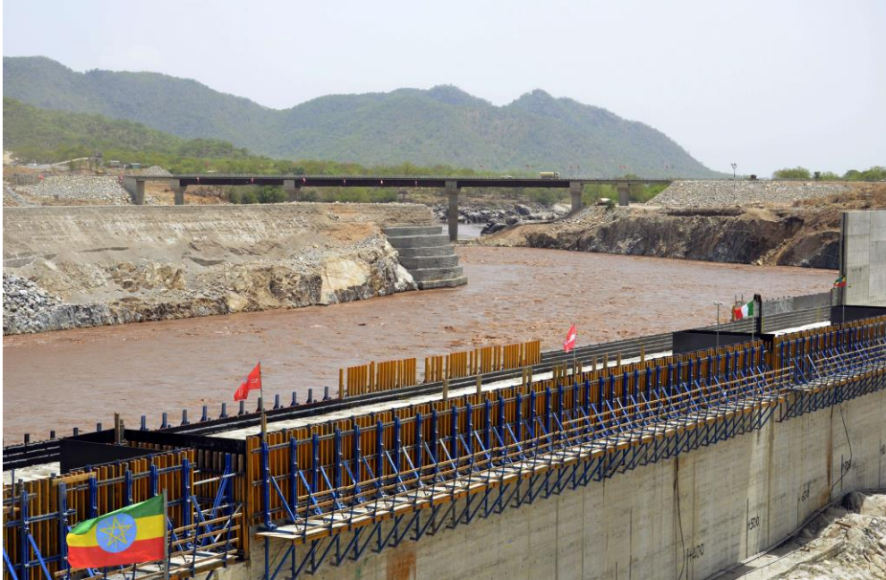
Figure 5-2: Picture showing construction of Ethiopian Grand Dam (Daily news Egypt, 2014)
