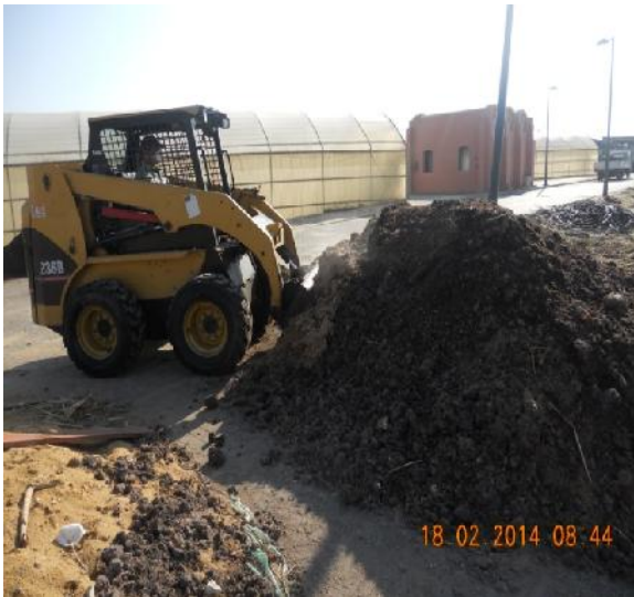
Figure 3.18. Mixing of compost windrows
