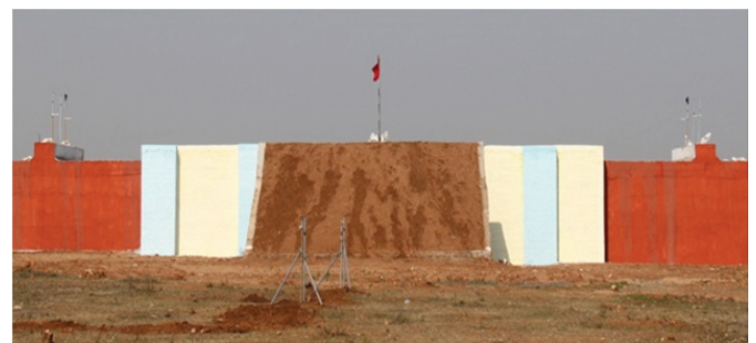
Figure 10. Deployment of Sensors in the field.
