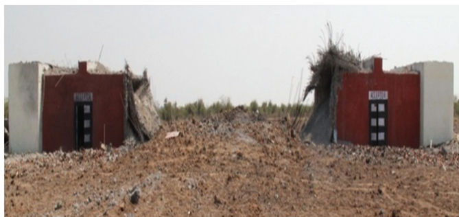
Figure 11. Structure after the blast.
