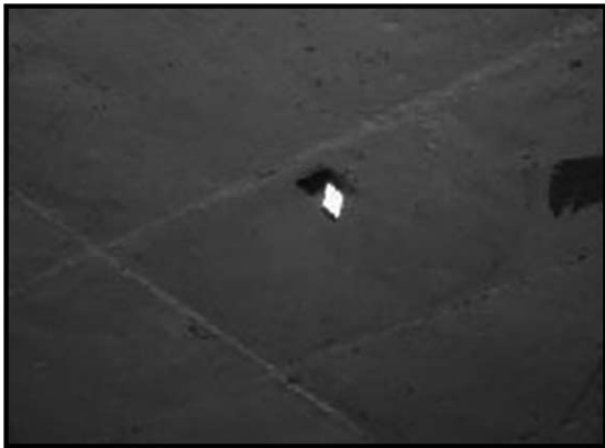
Figure 8. Arrangement for target to measure deflection of roof.
