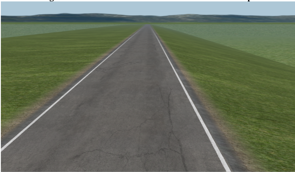
Figure 7. Straight road with a 3:1 side-slope
