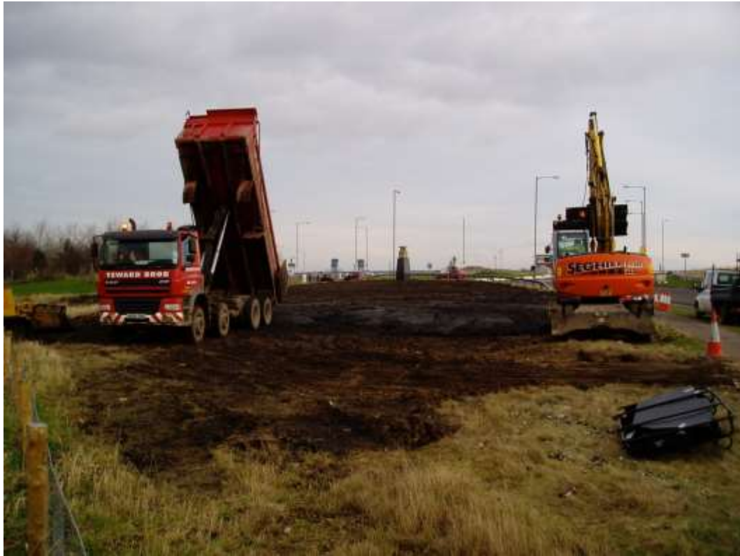
Figure 1. Material placement on restored brownfield site, Tees Barrage, Stockton-on-Tees, UK, February 2008.
