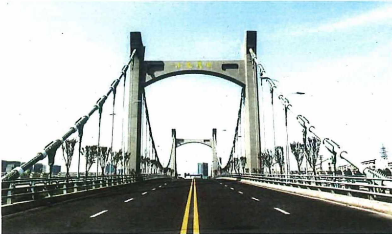
Fig. 13 Xiaolongwan Bridge in Nanjing (P.R. China)
