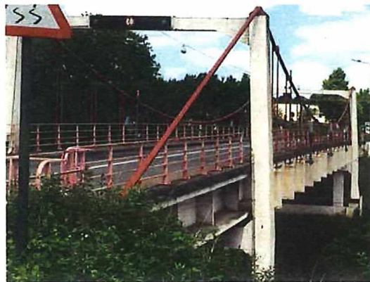
Fig. 9 First self-anchored suspension bridge (W13) (Photo: Luc Taerwe)
