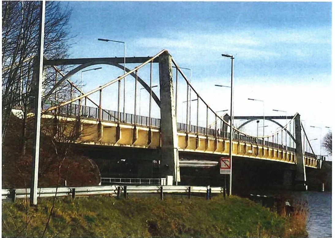
Fig. 11 Bridge W16 at Mariakerke (Photo: Luc Taerwe)
