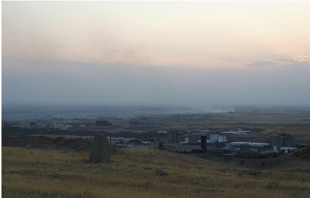
Figure 3.11 Oil storage tanks in study area, Erbil Province.
