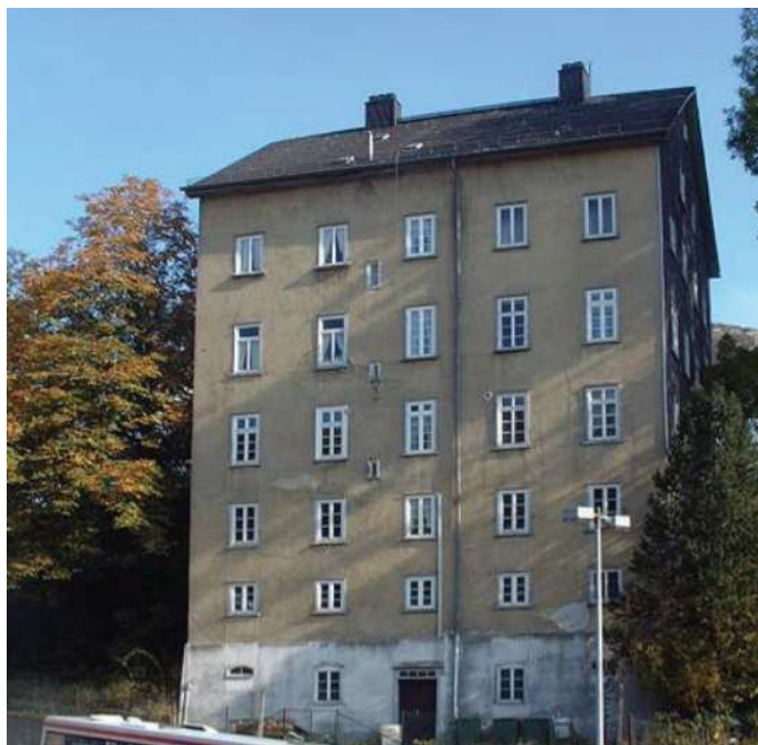
Figure 3: A residential building made in rammed earth, built in 1828, in Weilburg, Germany [2].
