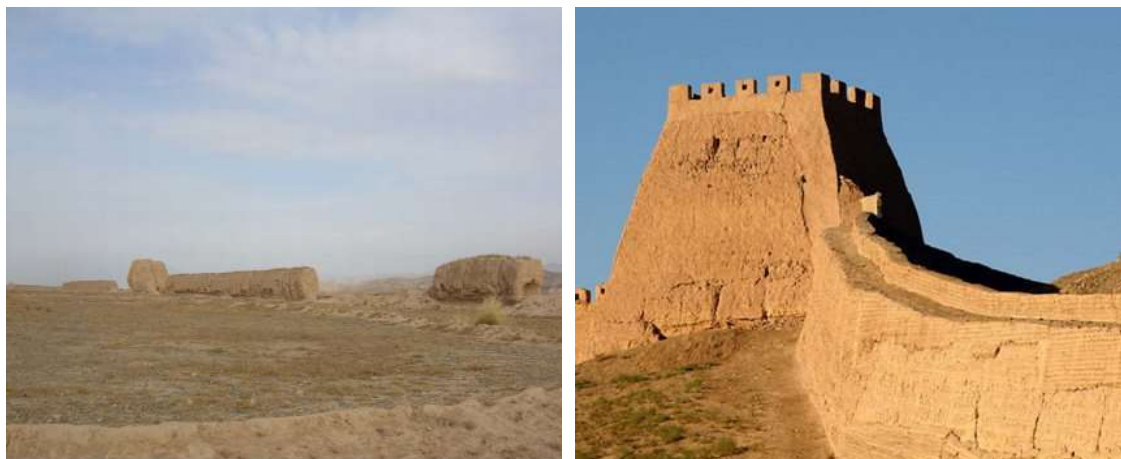
Figure 1: Parts of the Great Wall of China made on rammed earth [5], [6].
