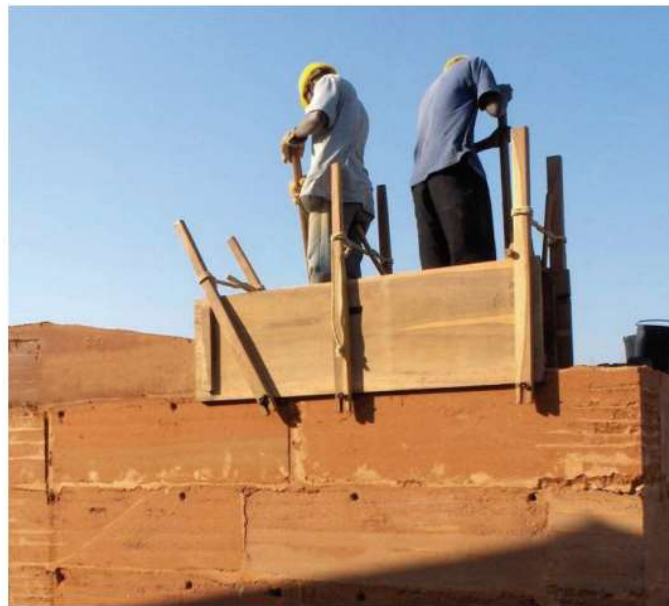
Figure 2: Manufacture of a rammed earth wall in Mumeno, Mozambique [4].
