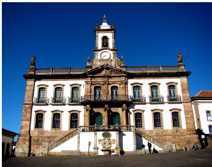
Figure 7: Old Town Hall and Prison of the city of Ouro Preto (Minas Gerais), built in rammed earth and stones [16].
