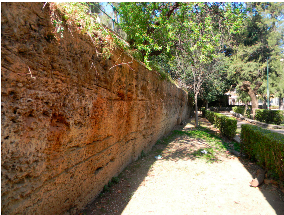
Figure 6. Ancient front of an historical opencast quarry cut in the calcarenite of Marsala and located in the current public garden 'Villa Garibaldi', within the Palermo town.
