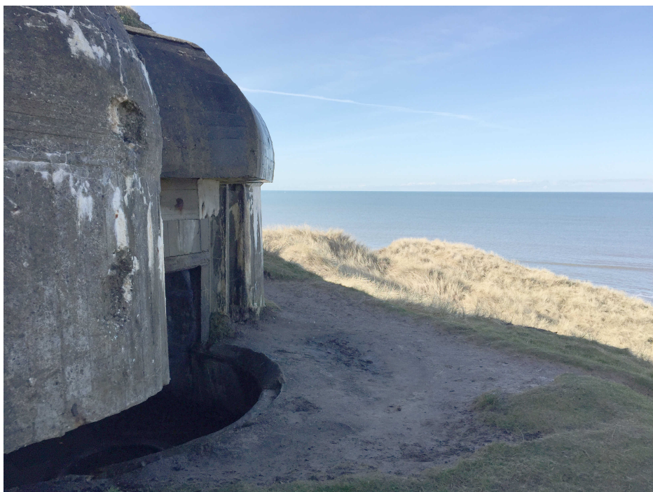
Complex of bunkers garrisoning the Danish coast. It is part of the defensive system of the Adriatic Wall built by the Germans from 1940 to 1944 to face the landing of the Allies.
