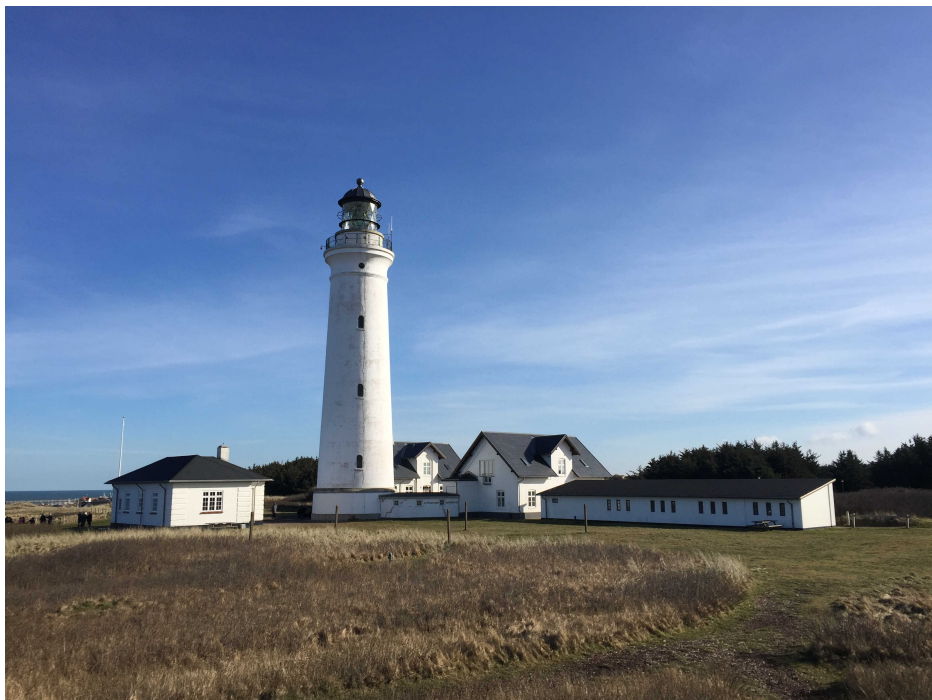
Hirtshals Fyr. Light and sound signal beacon built in 1868 on the northern coast of Denmark.
