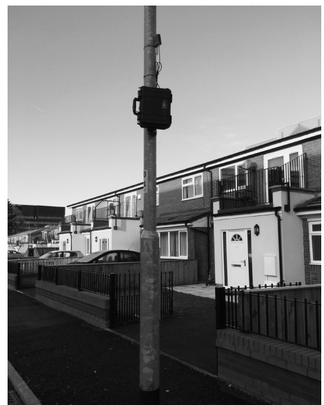
Figure 10.1.III-1 Black CAT Radar sensor positioned on a light pole
