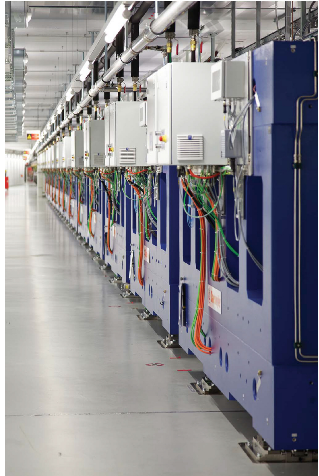
Figure 1: SwissFEL hard x-ray Undulator Aramis.
