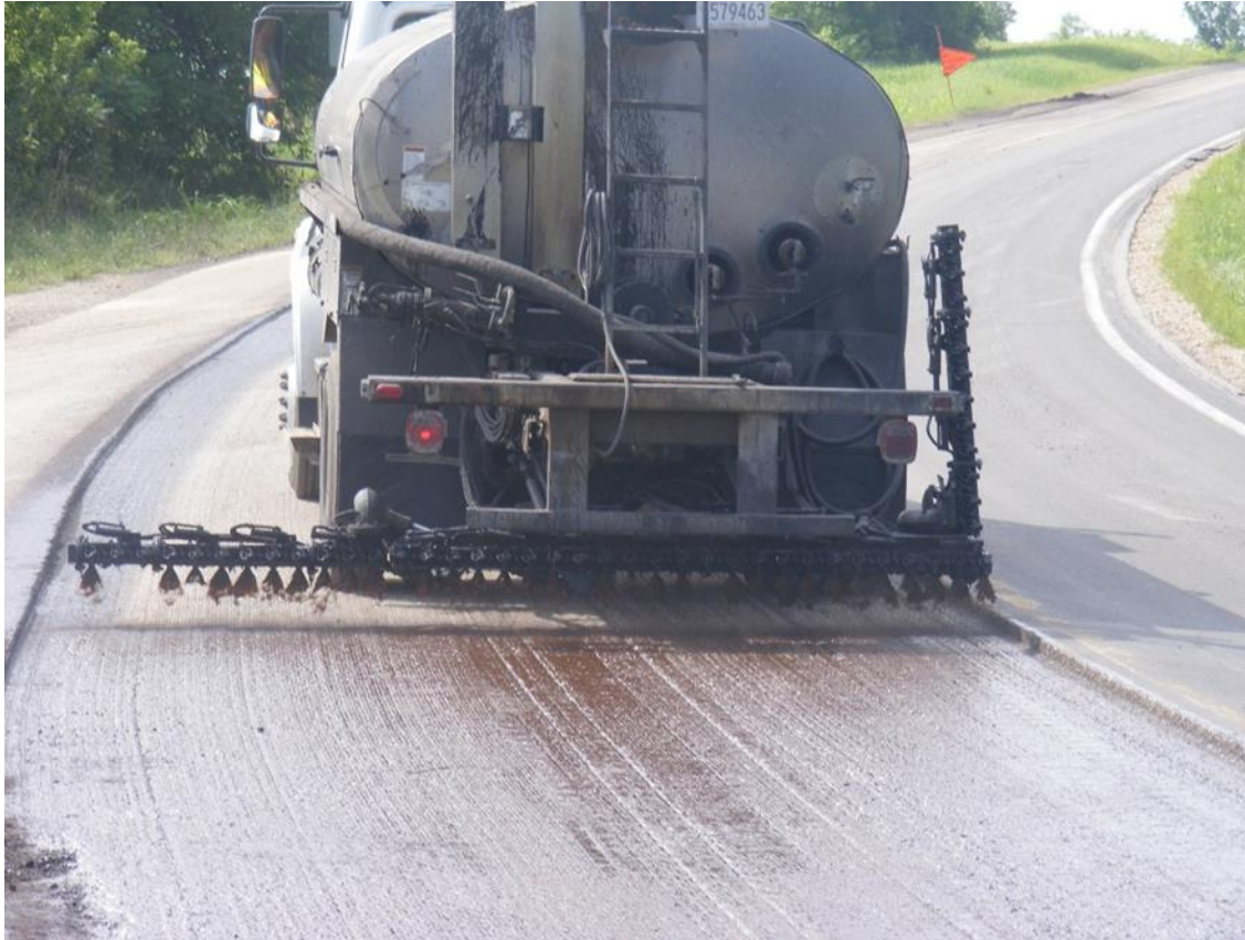
Figure 1.1 Tack Coat Application (Mealiff 2015)
