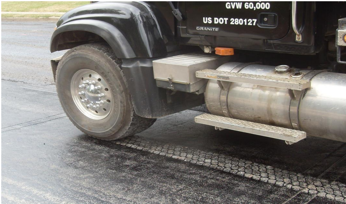
Figure 2.1 Tack Pickup by Truck Tire (Mealiff 2015)
