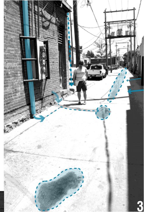
Figure 03. Alleyway Stormwater standing water during warm, sunny, summer afternoon (Krehbiel 2014)
