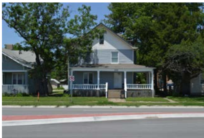
Figure 5: House D is at 1116 Bluemont Avenue (Prudenti 2014)
