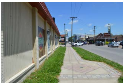
Figure 5: Concrete Pavers Introduced, Using Material Change To Define Business District
