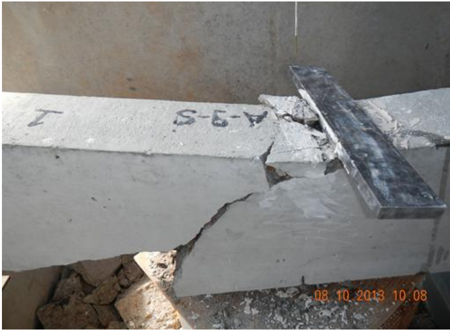
Figure H.57 Beam End A9-S Failure
