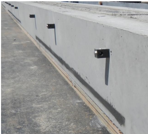
Figure 9.15 LSI Device Mounting Instrumentation
