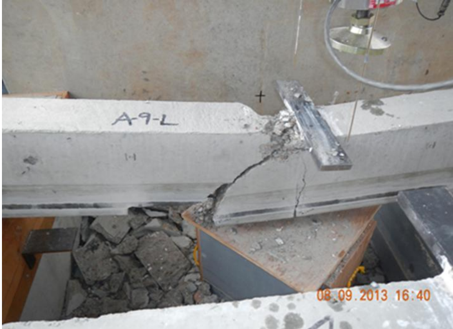
Figure H.27 Beam End A9-L Failure
