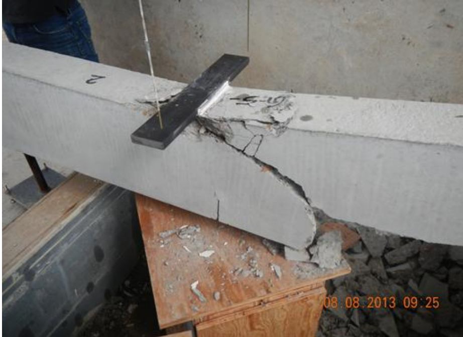
Figure H.104 Beam End G5-S Failure
