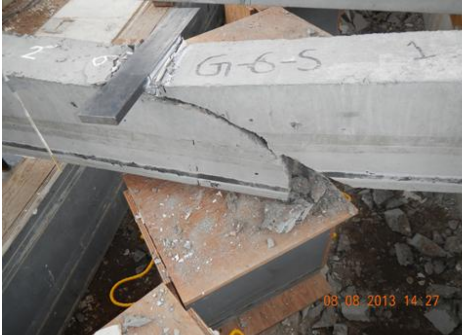
Figure H.107 Beam End G6-S Failure
