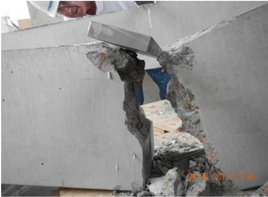
Figure H.155 Beam End I2-S Failure
