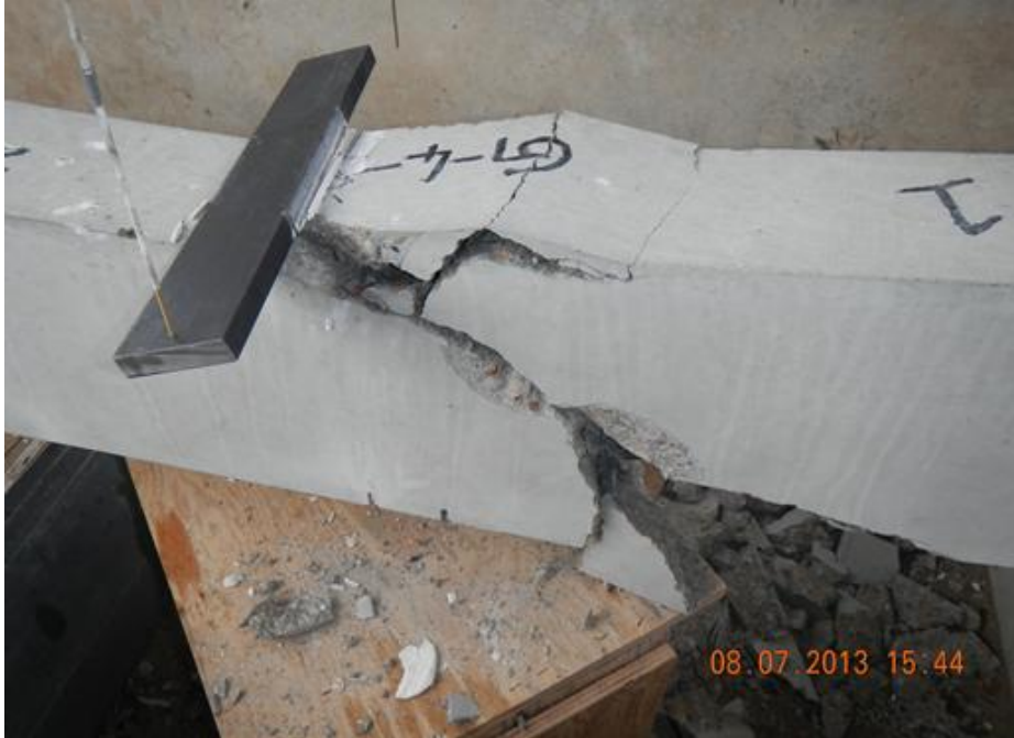
Figure H.101 Beam End G4-S Failure
