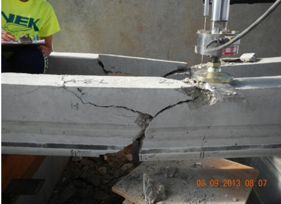
Figure H.24 Beam End A8-L Failure
