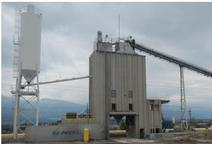
Figure 9.5 Concrete Mixing Plant at Stresscon, Inc.
