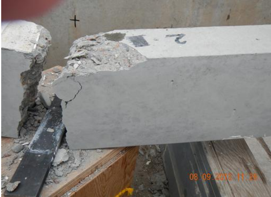
Figure H.51 Beam End A7-S Failure
