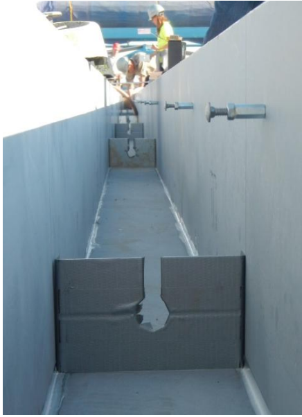
Figure 9.7 Crack Inducer Setup
