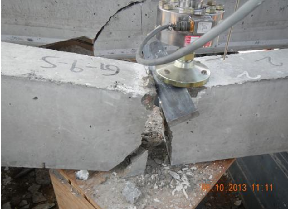
Figure H.116 Beam End G9-S Failure
