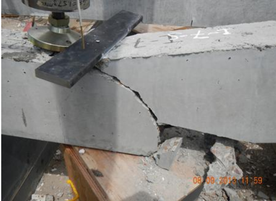
Figure H.170 Beam End I7-S Failure
