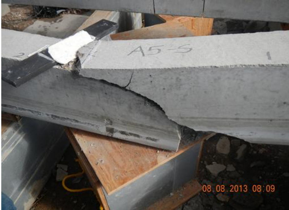
Figure H.45 Beam End A5-S Failure
