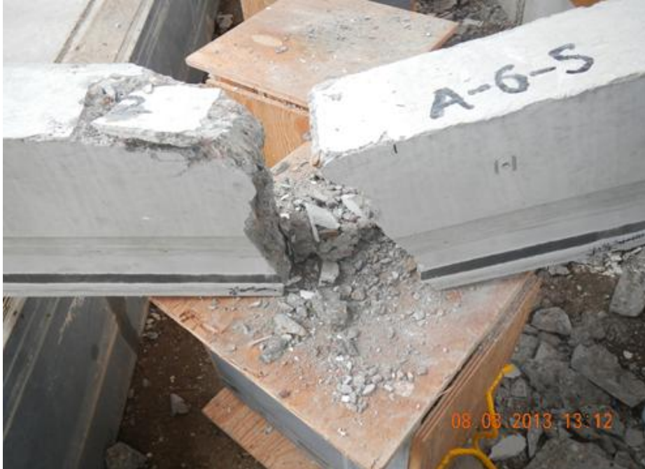
Figure H.48 Beam End A6-S Failure
