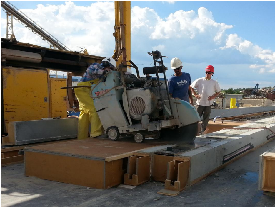
Figure 9.11 Saw Cutting of Flexural Beam Sections
