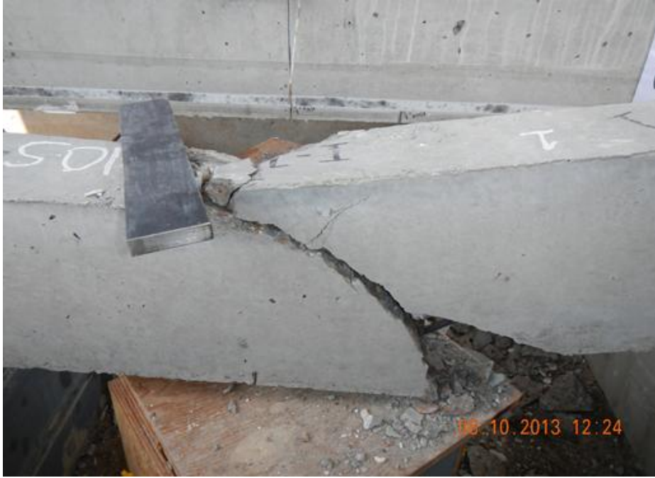
Figure H.179 Beam End I10-S Failure
