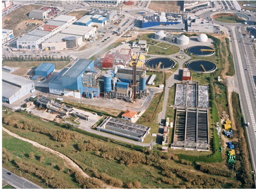
Figure 2.2. Aerial view of Mataró WWTP, location of the pilot plant
