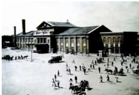
Figure 91. The Renaissance-style train station build by the Japanese in 1913, and demolished in 1994.
