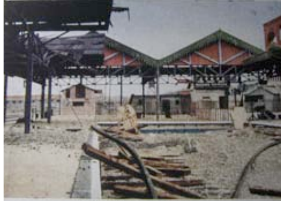
Figure 32. "A view of the Demolished North Station". 37
