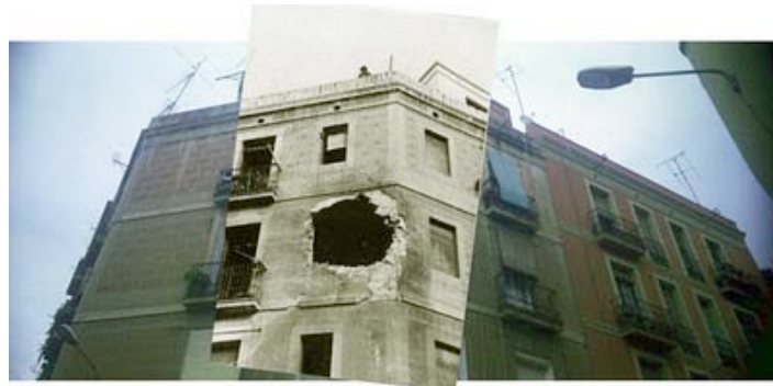
Figure 57. Rephotography combining an impact of mortar shell in a house from Barcelona Gracia neighborhood (11 Torres Street, corner with Tagamanent Street) during the first air raid over Barcelona during Spain's Civil War with a present photograph.
