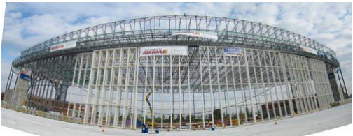
(b) Hangar in construction
