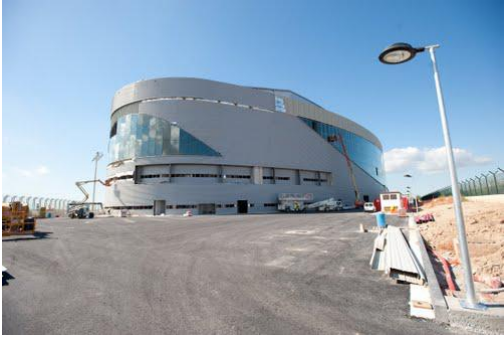
(c) Hangar finished
